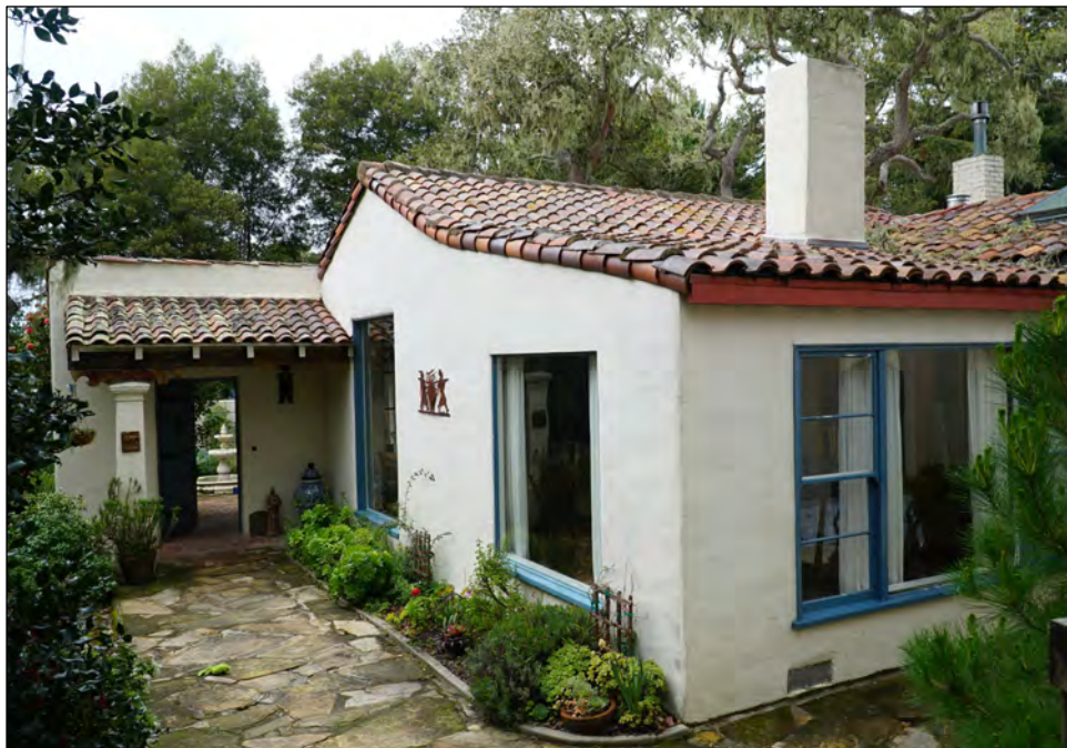
Figure 1. Looking northwest toward courtyard and south and east sides of house, 3/26/19.
