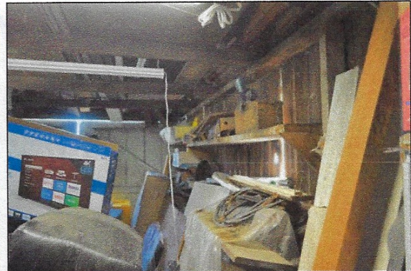
Figures 3 and 4. Left image details the shed-roofed addition to the south elevation. Note the sagging roof members and leaning walls. Right image details the garage interior's east wall, looking north, showing inadequate vertical and lateral support of the east wall.
