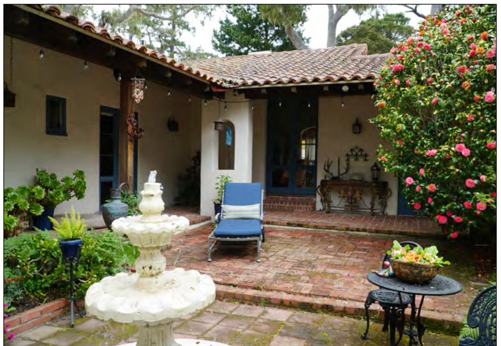
Figure 4. Looking northeast at south and west sides of courtyard designed by Clarence A. Tantau, 3/26/19.
