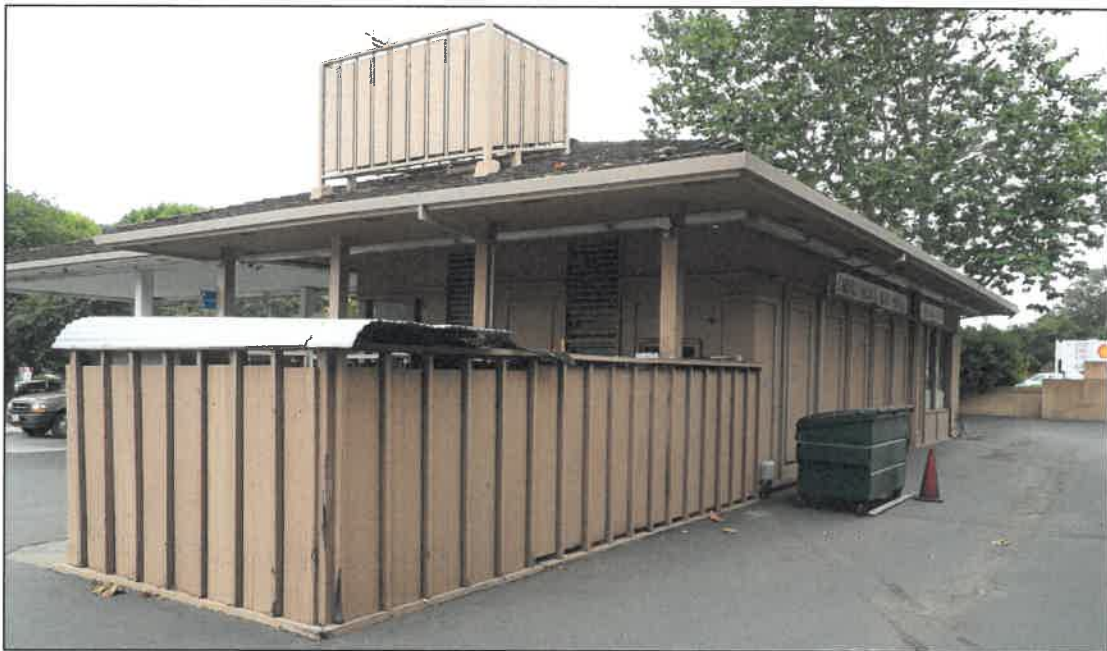
Figure 12. Looking southwest at east and north sides of Block 5, 19 August 2019.
