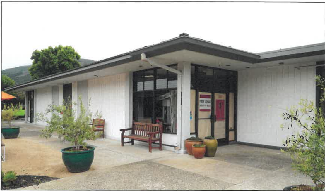
Figure 5. Looking southeast at north side of 1981 section of Block 2, 19 August 2019.
