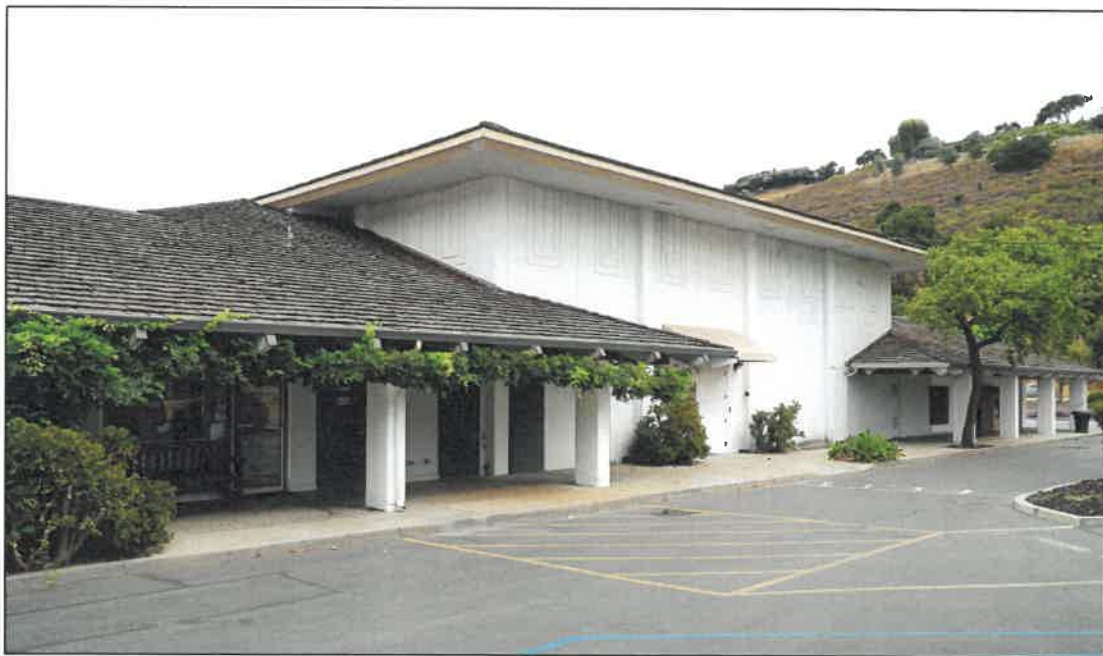
Figure 8. Looking northwest at east side of Block 3, 19 August 2019.
