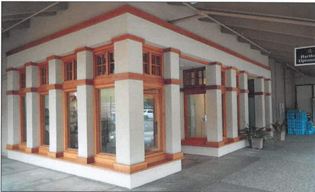
Figure 14. Looking southwest at two shops in Block 1, 19 August 2019. Their original appearance may be seen in Figure 13. The exteriors were radically altered about 1994.
