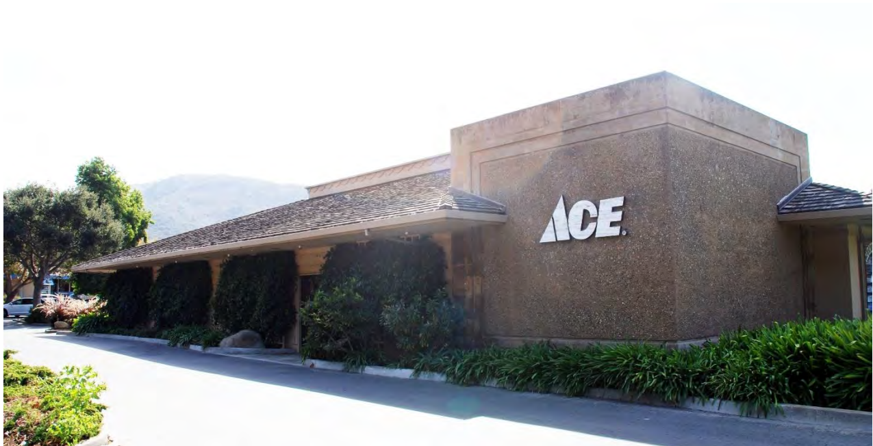
Figure 6. Ace Hardware store (former Crocker-Citizens Bank), 2019, view southeast. Source: Page & Turnbull
