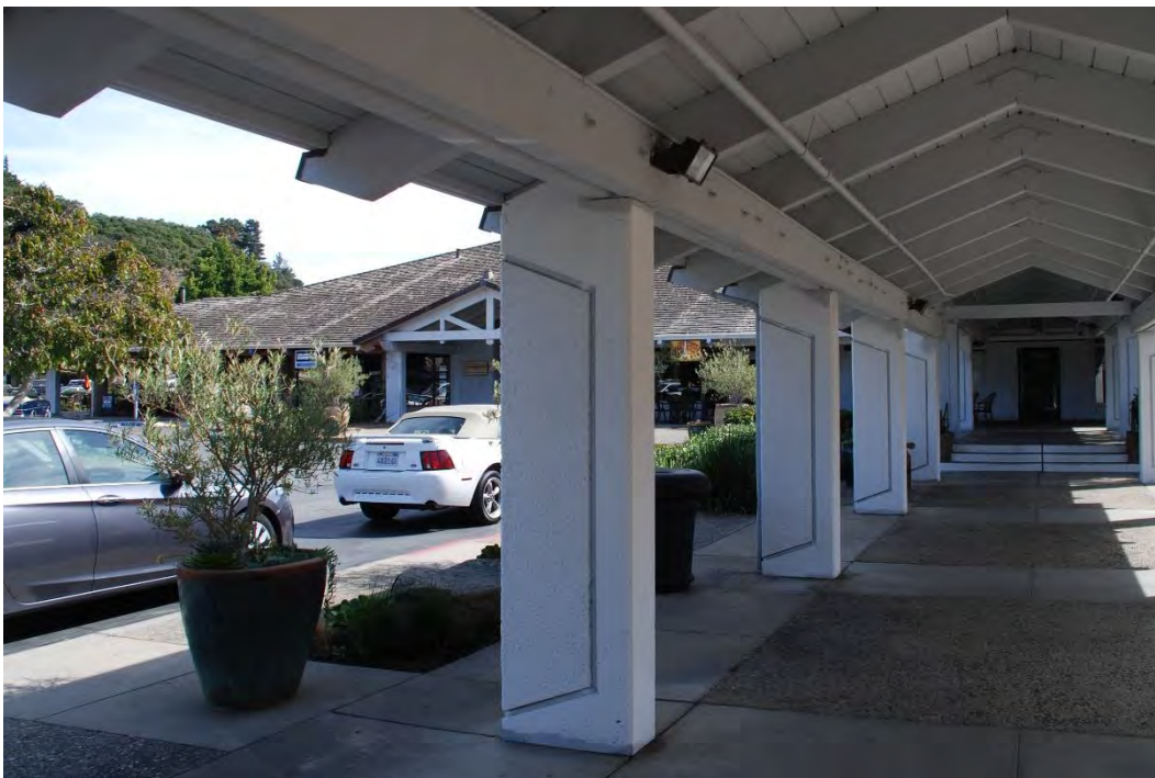
Figure 8. 2019 view of former cinema portion of Mid Valley Shopping Center, from covered walkway. Source: Page & Turnbull
