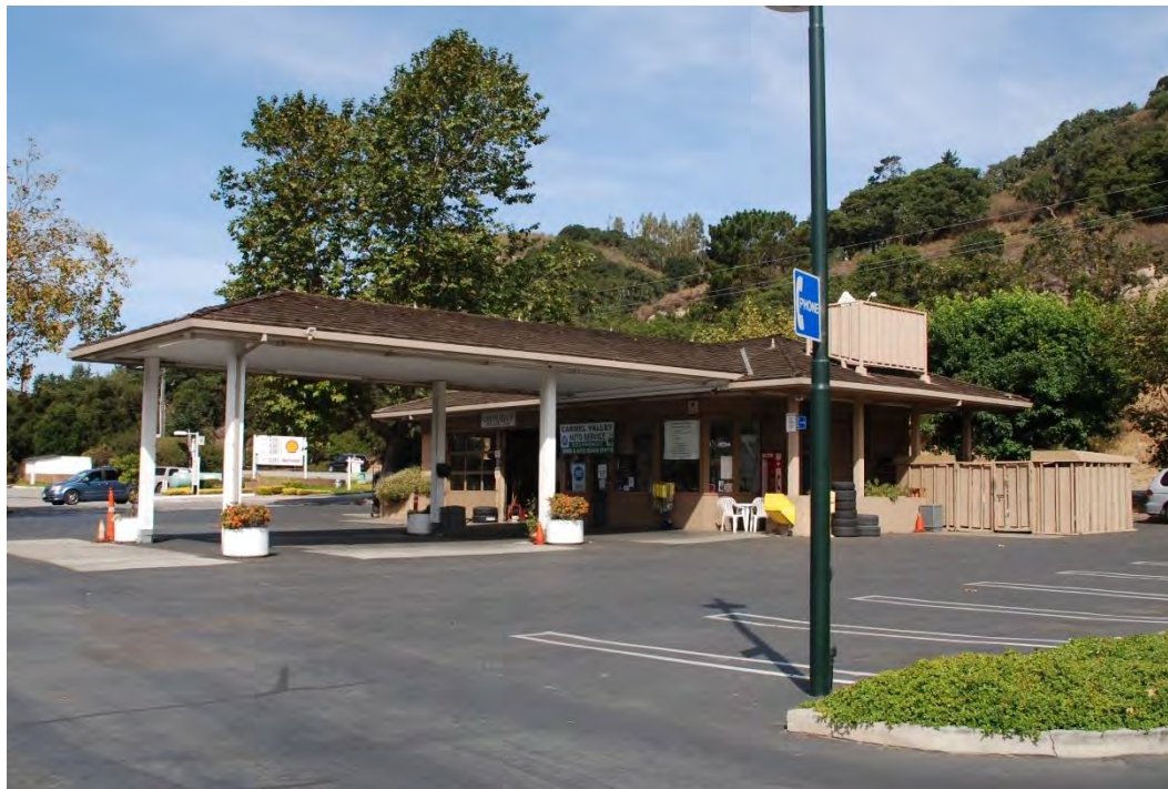
Figure 25. Building E, southwest and southeast façades, view northwest.
