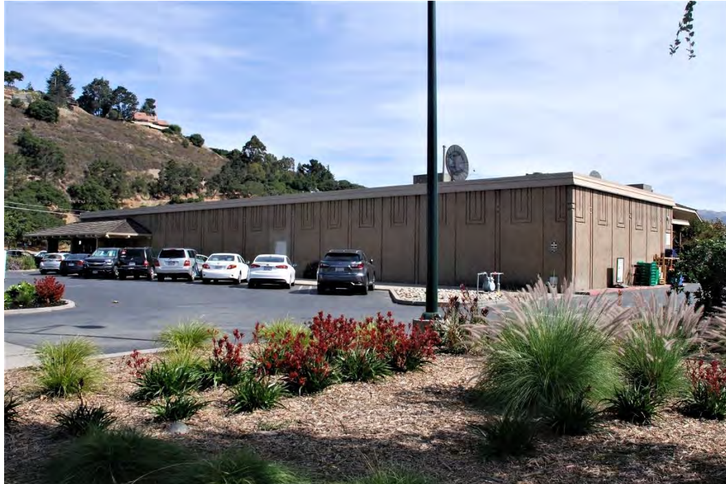
Figure 5. Building A, northwest façade and western portion of southwest façade, view northeast. Note intaglio wrapping around to rear of building.
