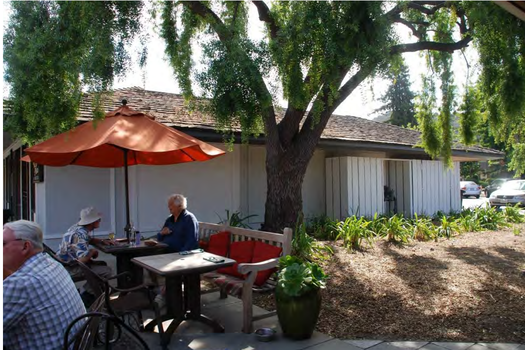
Figure 10. Building B, northwest façade, view southeast.
