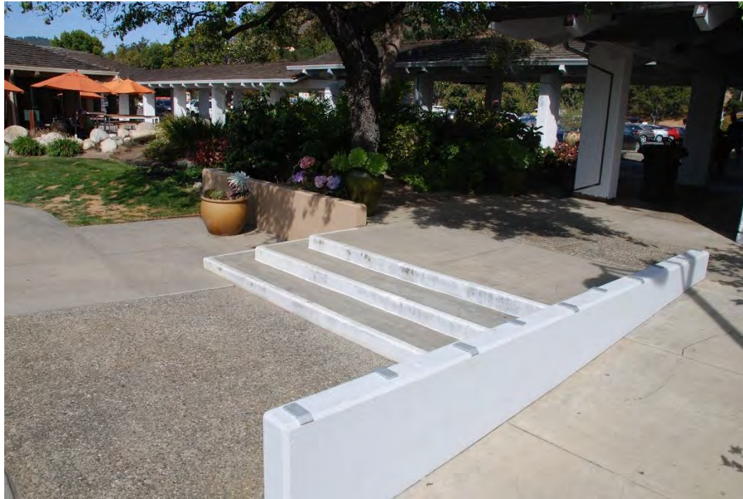
Figure 29. Courtyard between Buildings A, B, and C, view northwest toward covered walkway.
