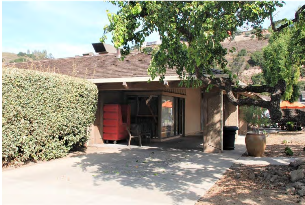
Figure 8. Building A, view northeast across southeast façade.
