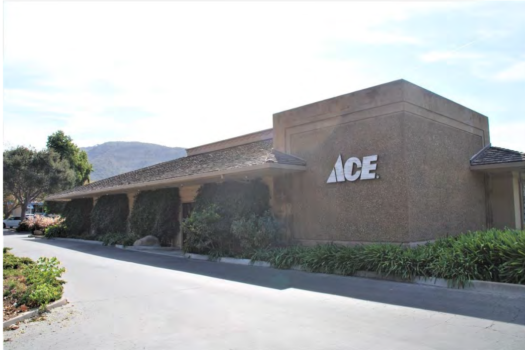
Figure 22. Building D, northeast façade, view southeast.
