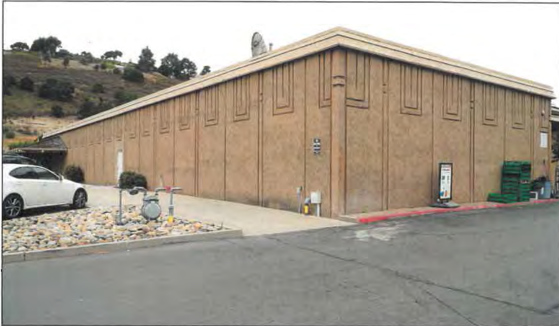
Figure 3. Looking northeast at west and south sides of Safeway, Block 1, 19 August 2019.
