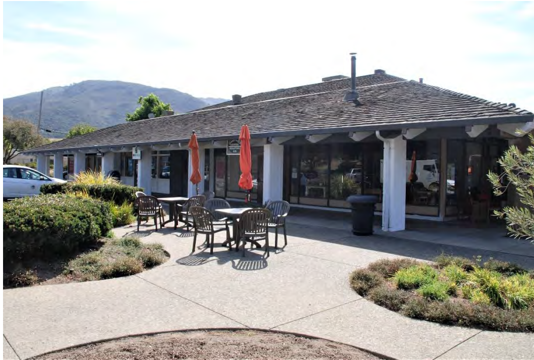
Figure 20. Building C, northeast façade, view southeast.
