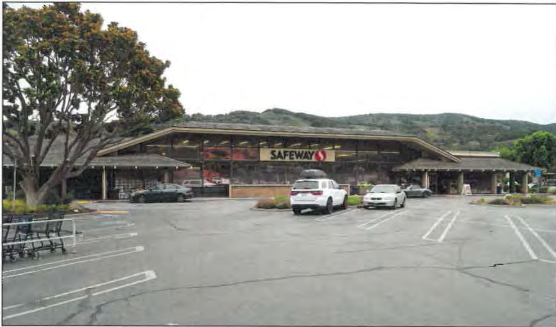
Figure 1. Looking southwest at north side of Block 1, 19 August 2019.
