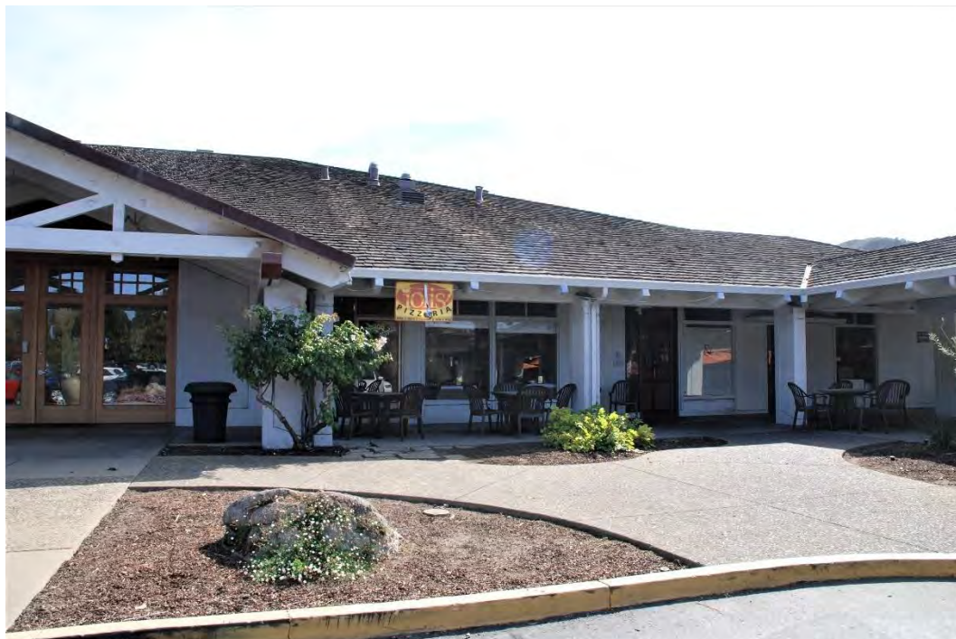
Figure 15. Building C, south portion of northwest façade, view southeast. Covered walkway attaches to Building C roof at right.
