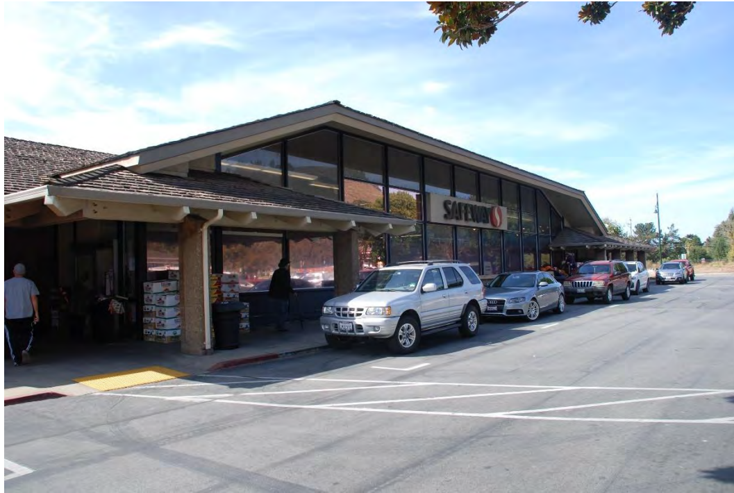
Figure 2. Building A, northeast façade of Safeway store, view southwest.
