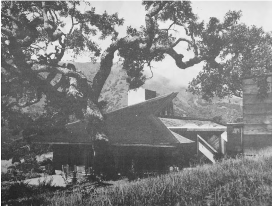
Figure 50. Dodds Residence, Carmel Valley, designed 1960-1961. Source: Architecture of the Monterey Peninsula .
