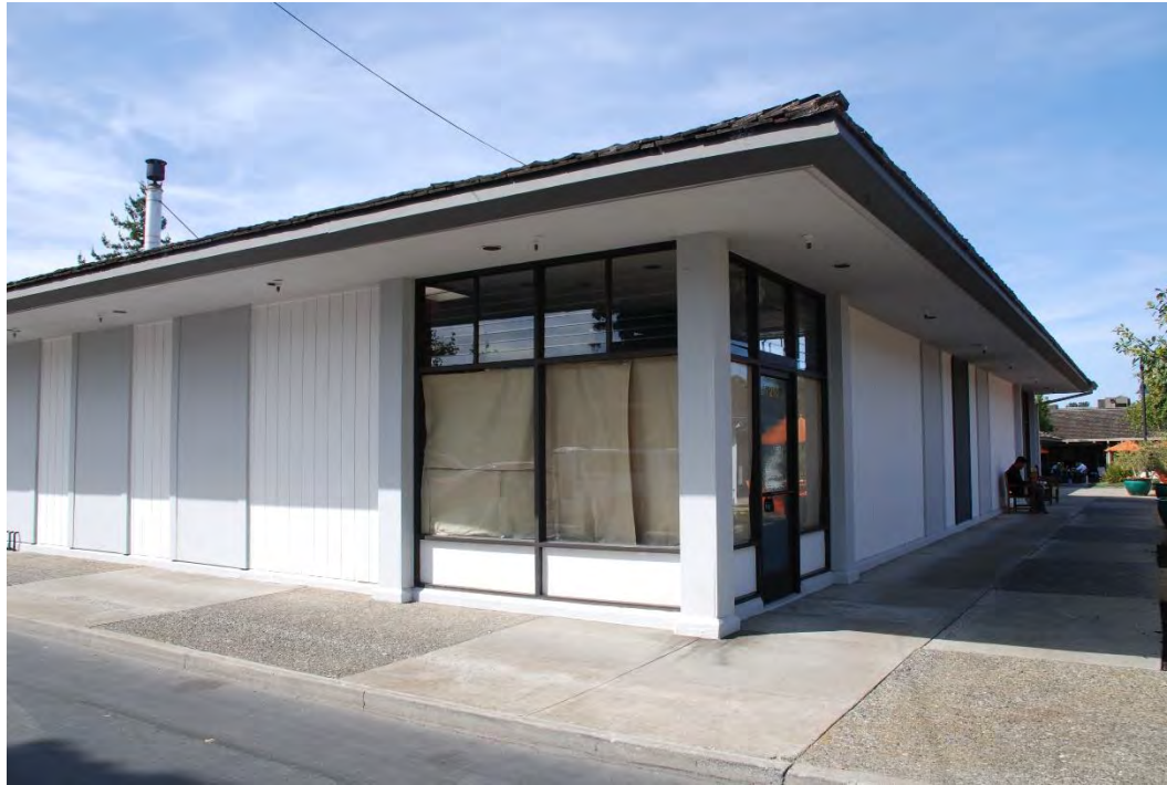
Figure 13. Building B, east portion of southeast façade and northeast façades, view west.
