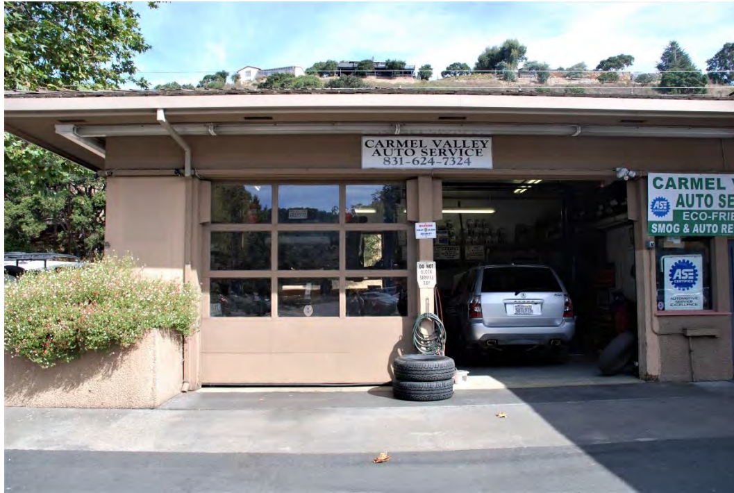
Figure 26. Building E, roll-up doors at west side of southwest façade, view northeast.
