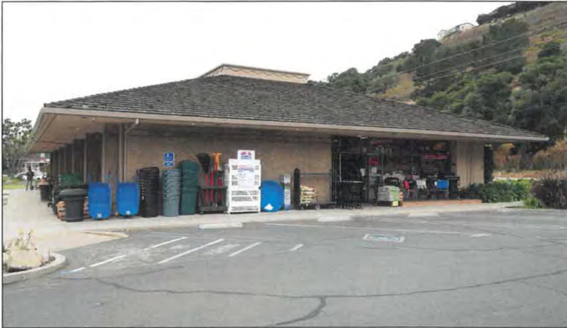
Figure 9. Looking northwest at south and east sides of Block 4, 19 August 2019.
