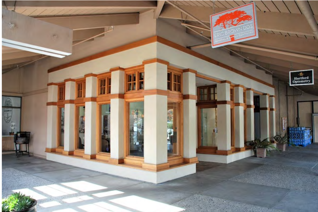
Figure 3. Building A, Two storefronts to immediate southeast of Safeway, view southwest.
