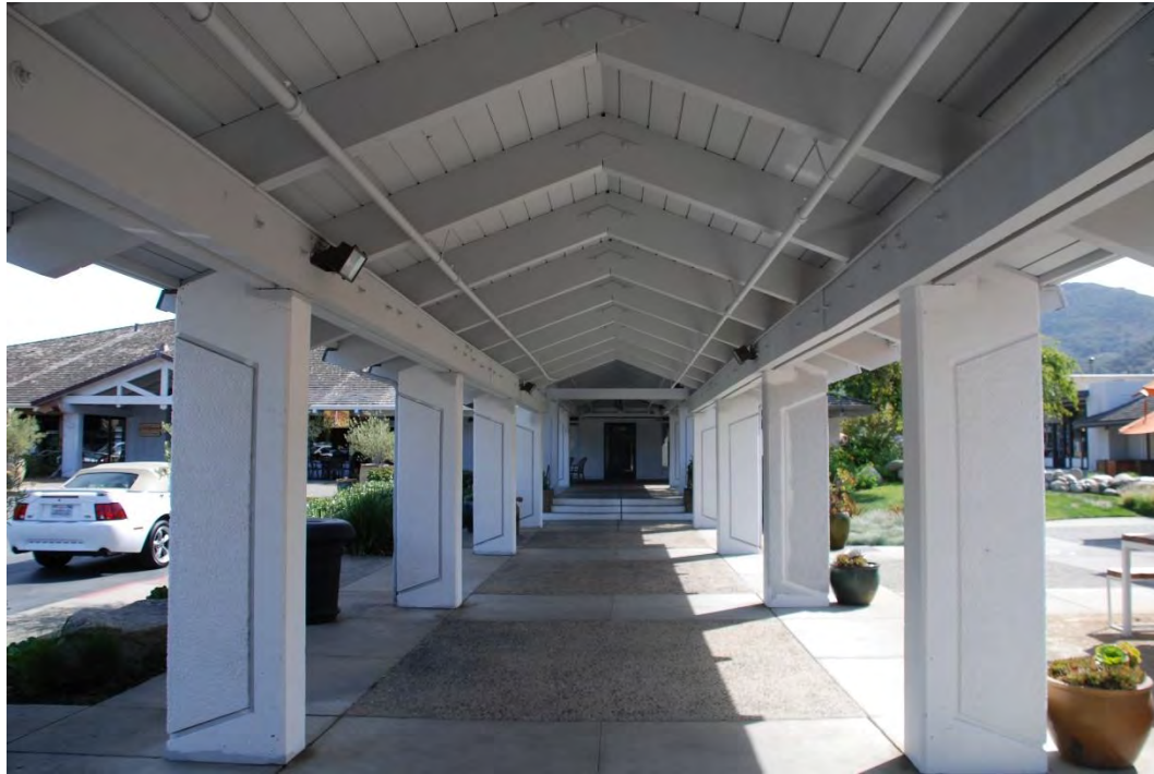
Figure 31. Covered walkway between Buildings A and C, view southeast.
