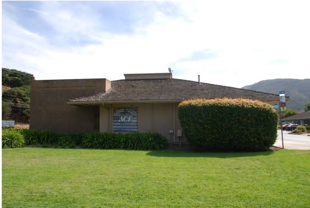
Figure 23. Building D, northwest façade, view southeast.
