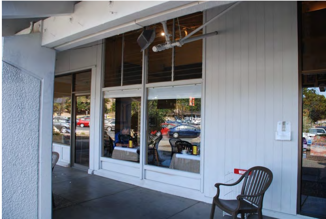
Figure 16. Storefronts at southwest end of Building C, view northeast.
