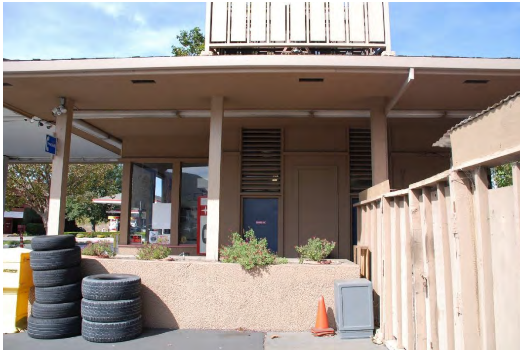
Figure 28. Building E, southeast façade, view northwest.
