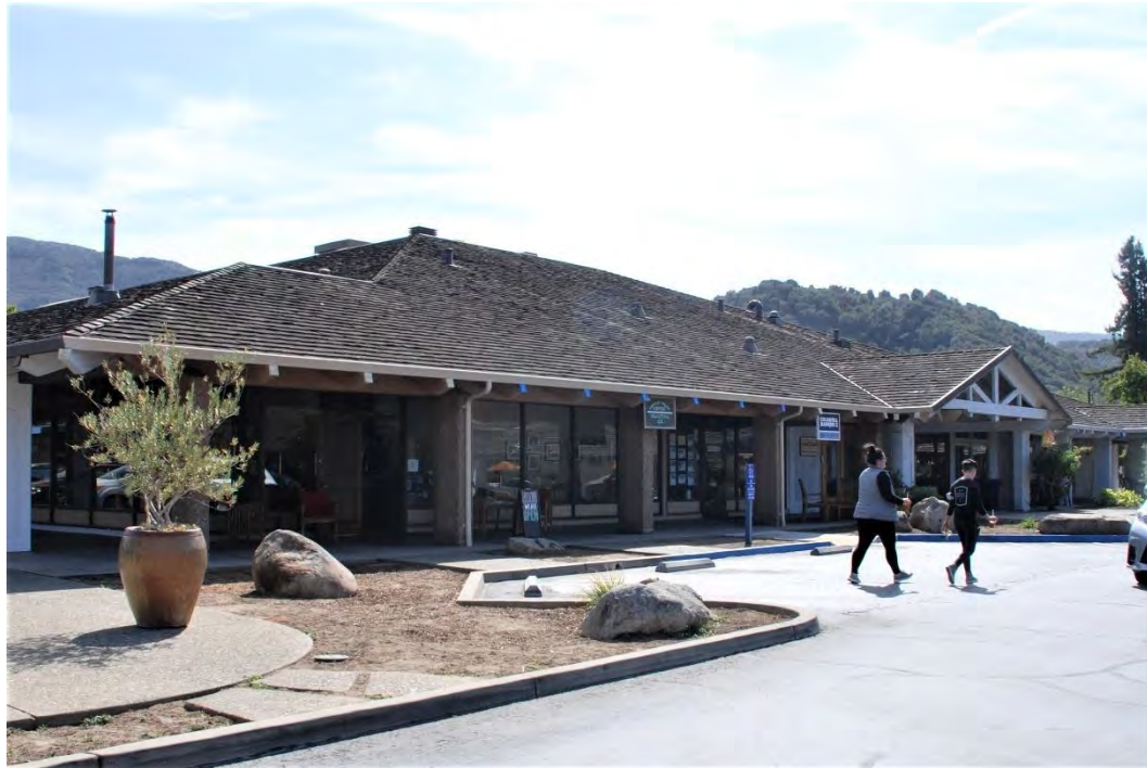
Figure 14. Building C, northwest façade, view south.
