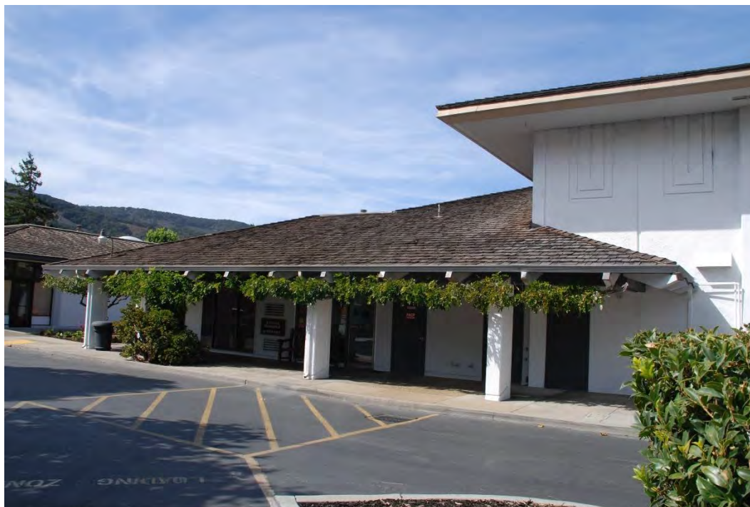
Figure 18. Building C, south portion of southeast façade, view west.
