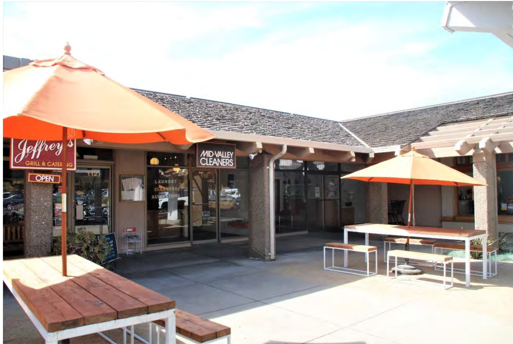
Figure 4. Building A, northeast façade of southeast wing, view southwest. The edge of the covered walkway is visible at the upper right.
