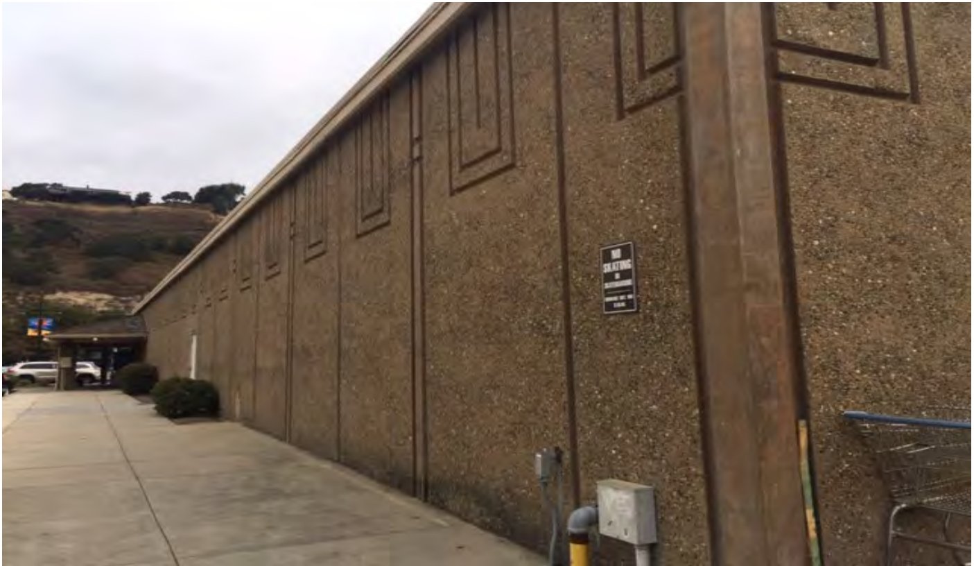
Figure 4. The blank wall along the west elevation
