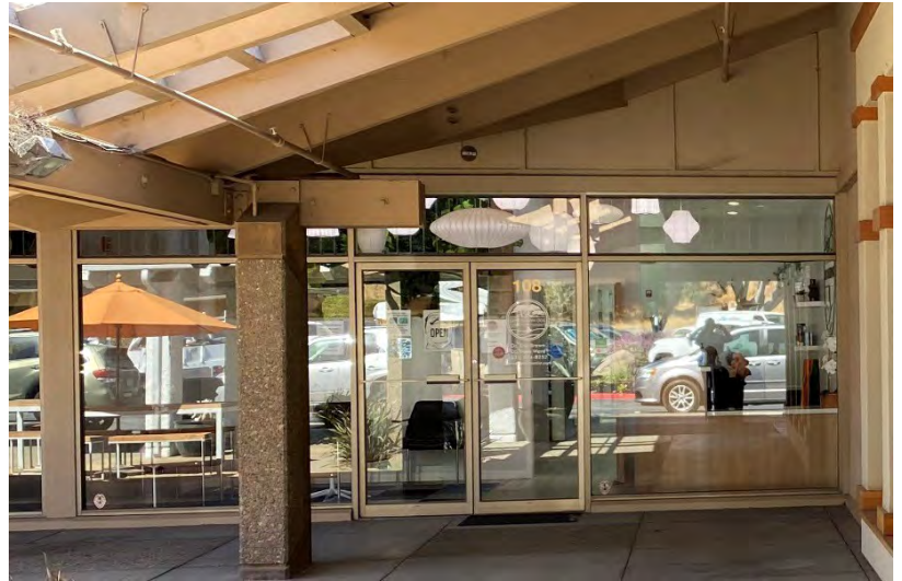
Figure 11. North elevation of Shop
