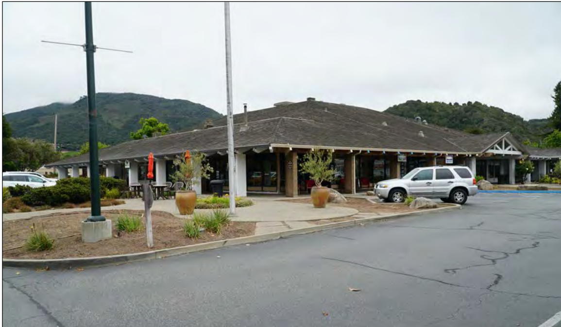
Figure 8. Looking southeast at north and west sides of Building B-2, 19 August 2019.
