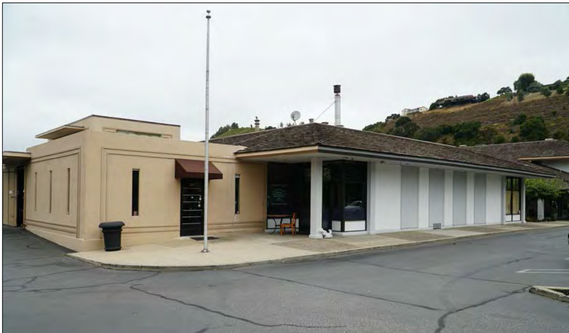
Figure 7. Looking northwest at south and east sides of 1981 and 1982 sections of Building C, 19 August 2019.
