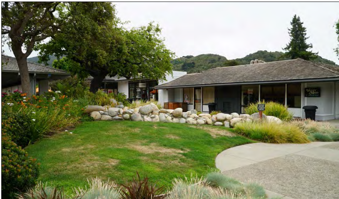
Figure 5. Looking southeast at north side of Building C.
