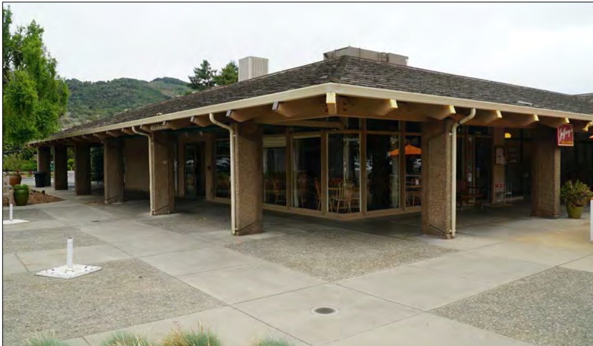
Figure 3. Looking southwest at east and north sides of Building B-1, 19 August 2019.
