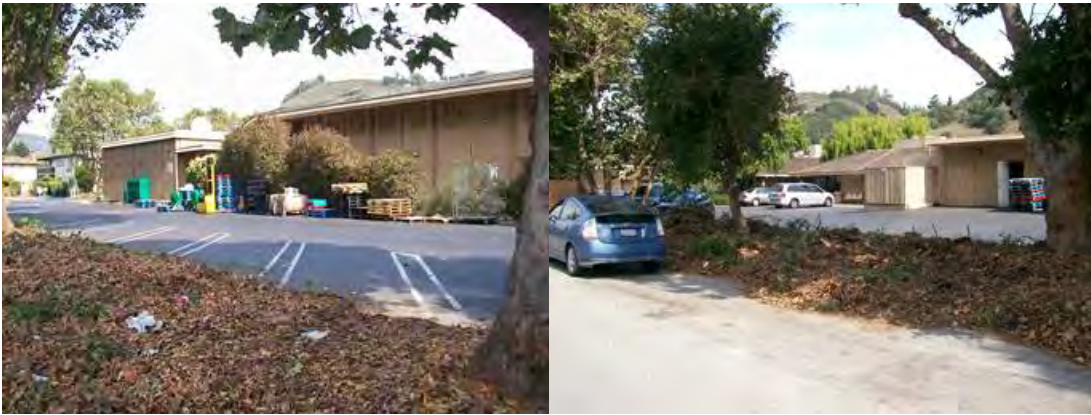
Mid Valley Garden HOA faces the back-side of the one-block long shopping center.
