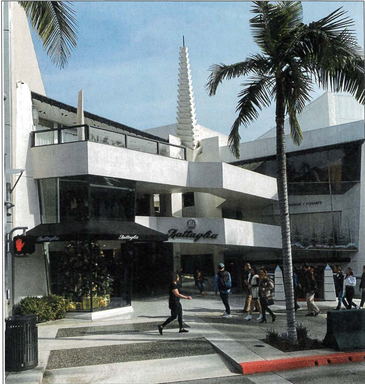
Figure 1. Frank Lloyd Wright, Anderton Court Shops, Rodeo Drive, Beverly Hills, California. The small shopping center opened in 1952 and was added to the National Register of Historic Places in 2004.
