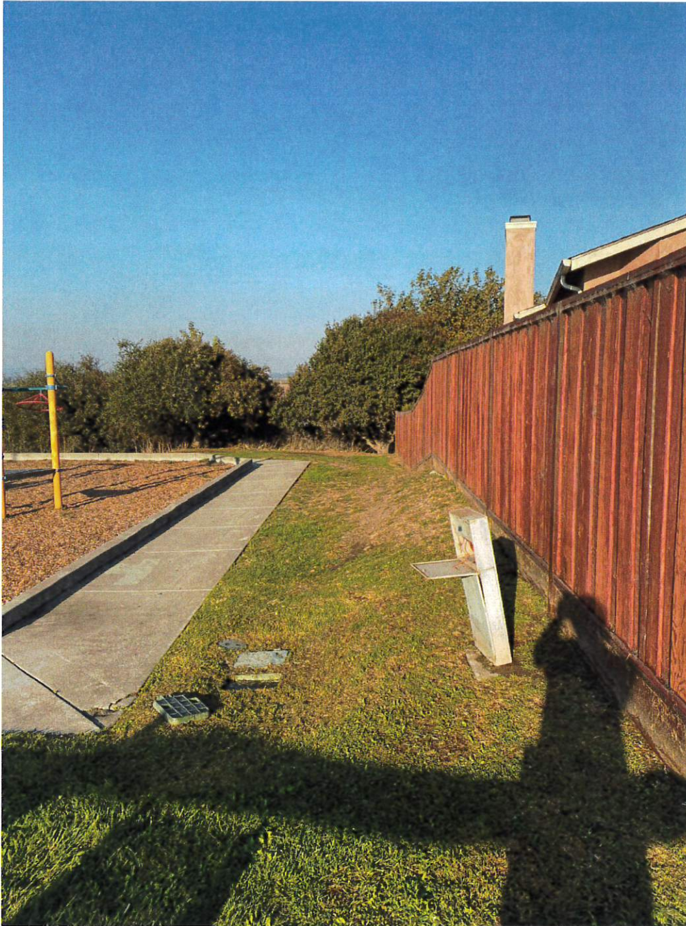
View along southeast side of parcel looking northeast. Note position of sprinkler control box approximately 12" from walkway.
