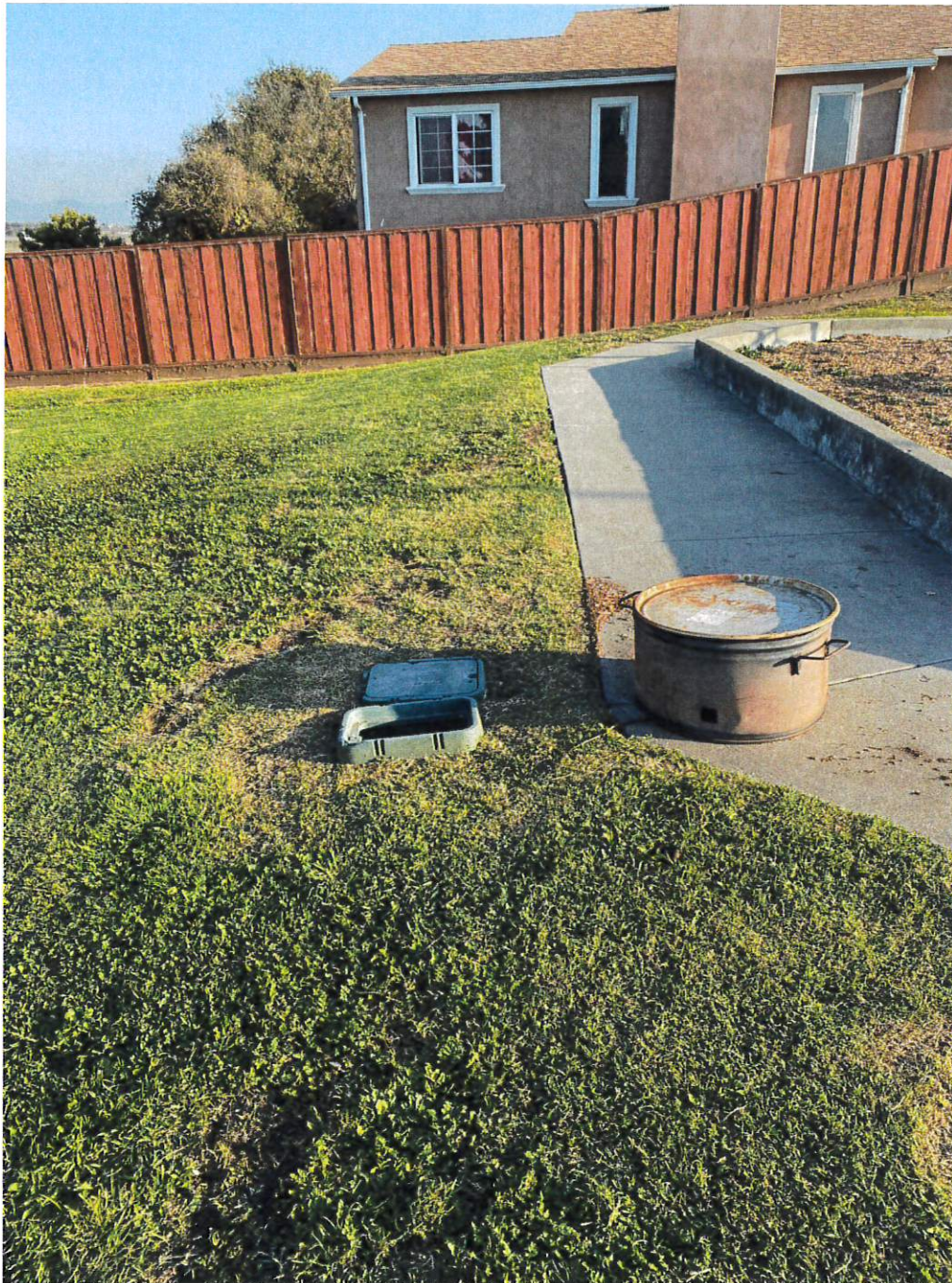
View of walkway at northeast side of play structure with irrigation box approximately 12" outside of walkway.
