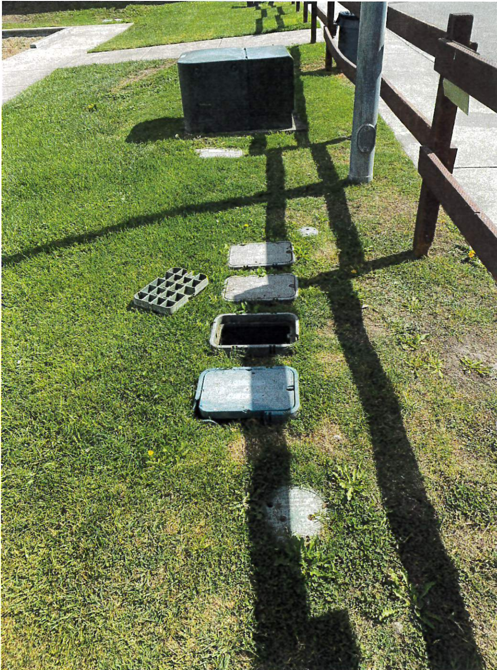
Irrigation control boxes, street light pole, and utility box along southwest edge of parcel between the play structure and sidewalk.
