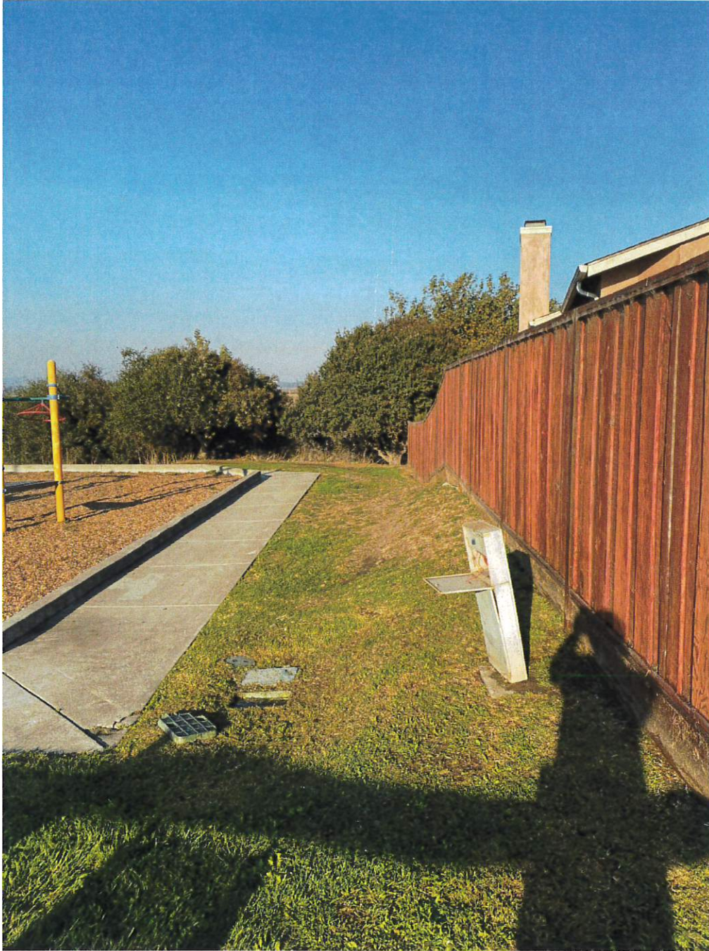
View along southeast side of parcel looking northeast. Note position of sprinkler control box approximately 12" from walkway.
