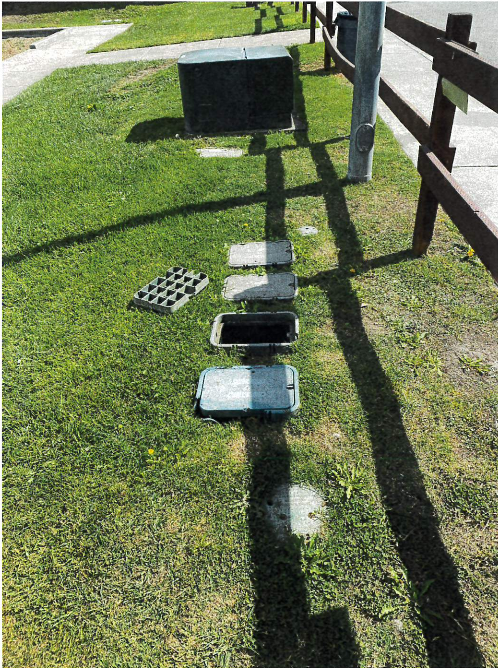
Irrigation control boxes, street light pole, and utility box along southwest edge of parcel between the play structure and sidewalk.
