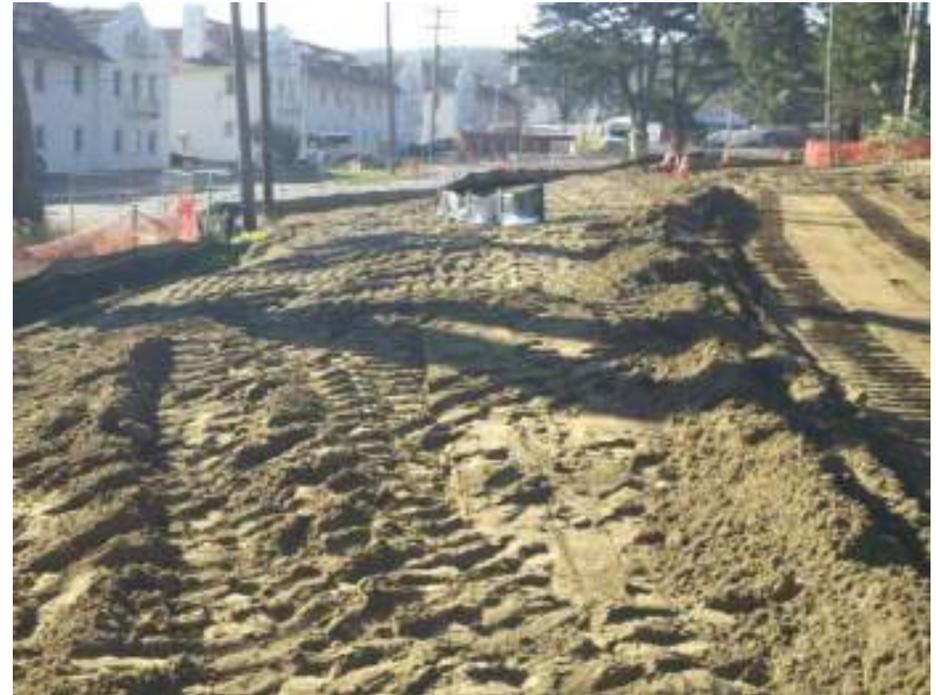
Heavy machinery was used to track walk these soils.
