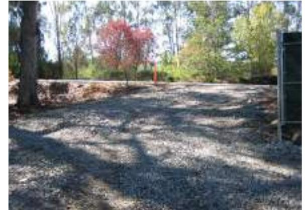
The contractors properly installed a stabilized construction roadway.
