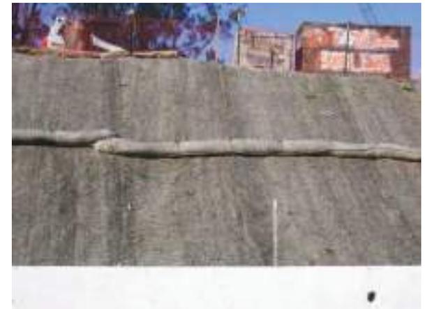
Jute netting with fiber rolls are installed to stabilize this steep slope along the roadway.
