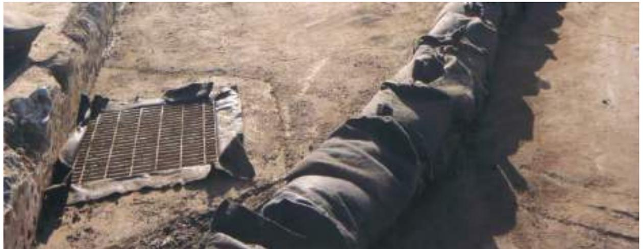
A gravel berm acts a sediment trap near a catch basin.
