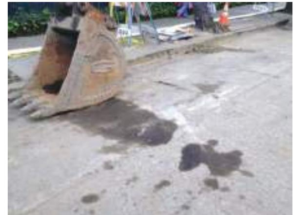
Minor oil spills need to be cleaned to prevent them from running into the storm drain system.
