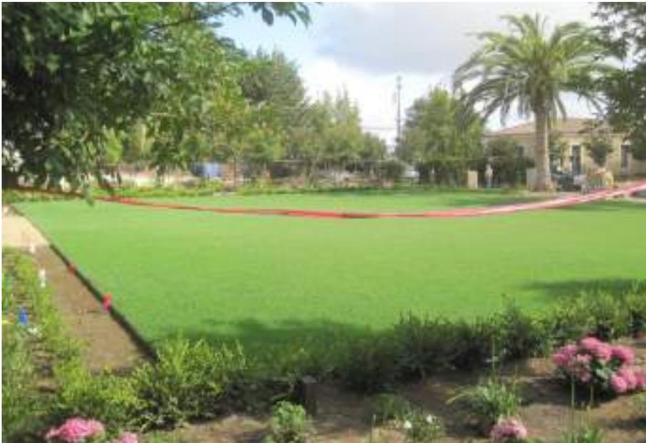
Sod is installed to provide permanent vegetation and erosion control.
