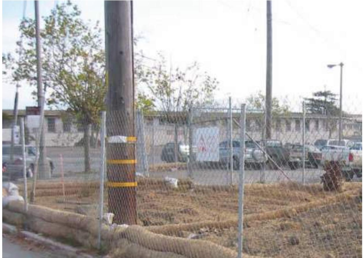
Erosion control blankets are being used to stabilize disturbed soil area.
