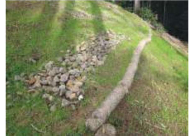
Fiber rolls are installed along a hillside to reduce erosion.
