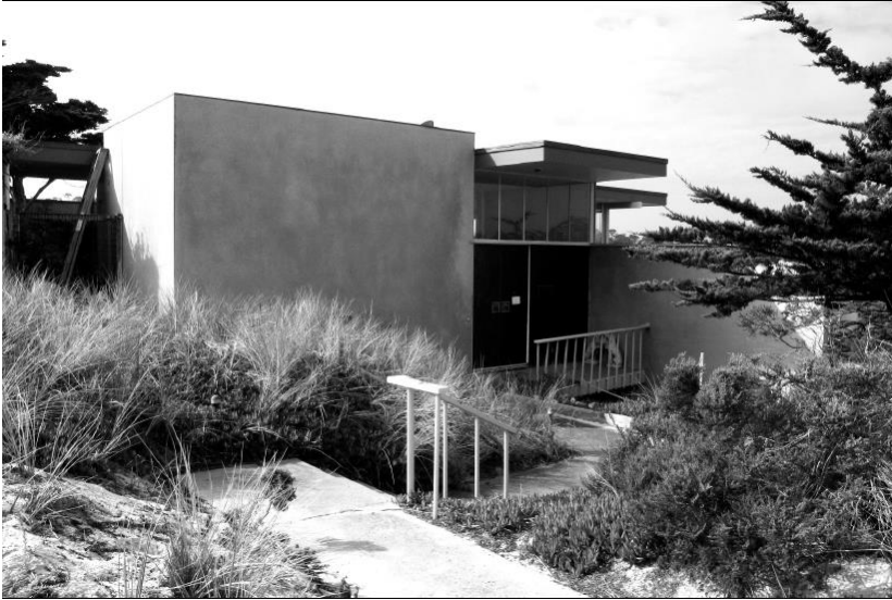
Photo 1 Kirk photo of building's north side, looking southwest, 5 October 2010.
