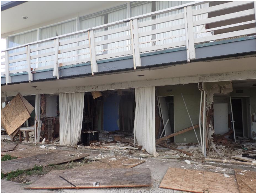
Photo 6 SWCA photo looking east from the lower level, west side.
