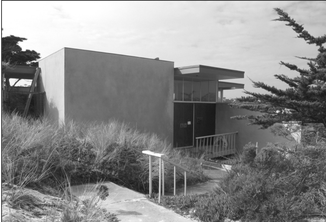
Figure 4.3-6. North elevation, looking southwest.
