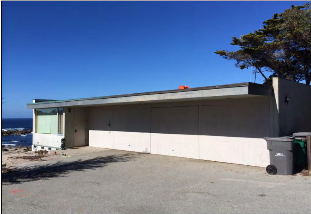
Figure 4.3-8. South elevation, looking northwest.
