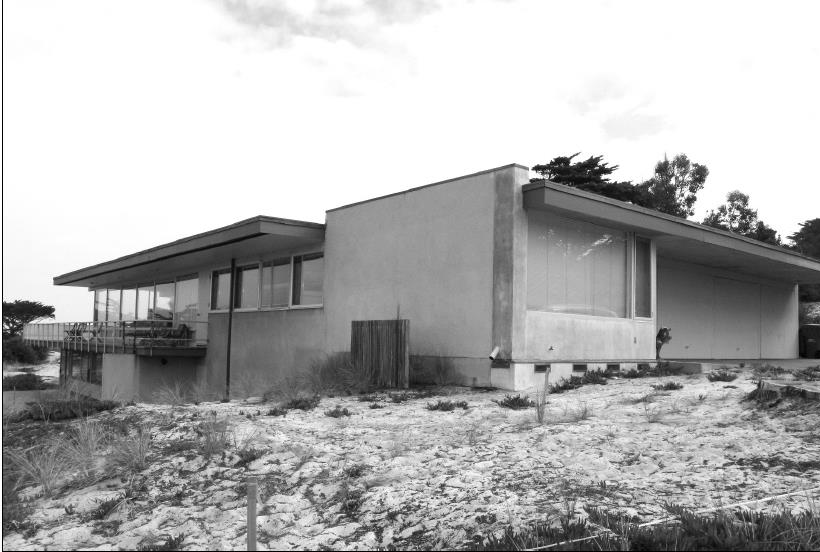
Photo 3 Kirk photo of southeast corner, looking northwest, 5 October 2010.
