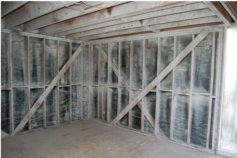
Photo 22 Interior view of upper level northeast corner.
