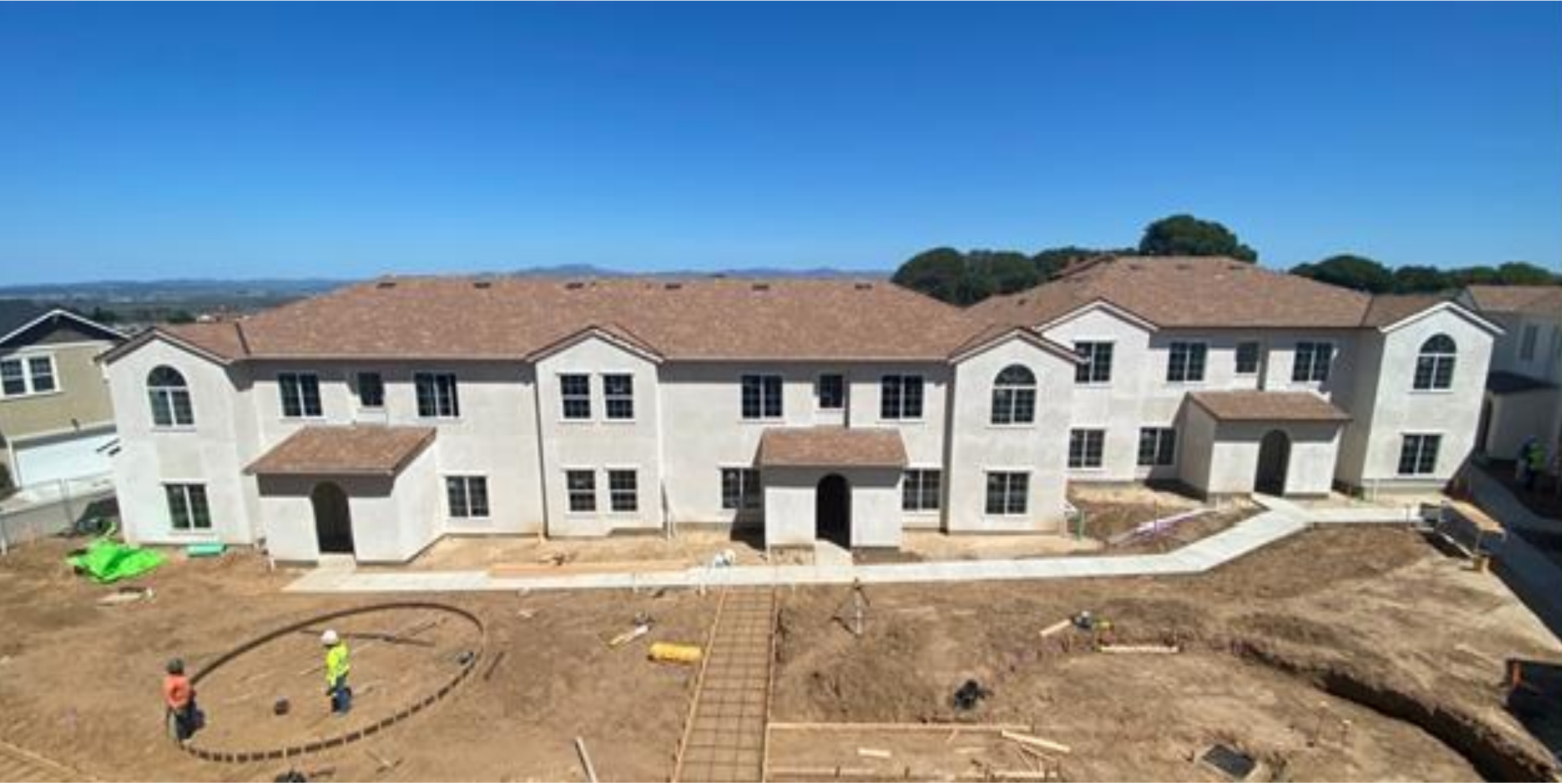
Alfred Diaz-Infante (formerly “East Garrison”) Apartments – currently under construction
