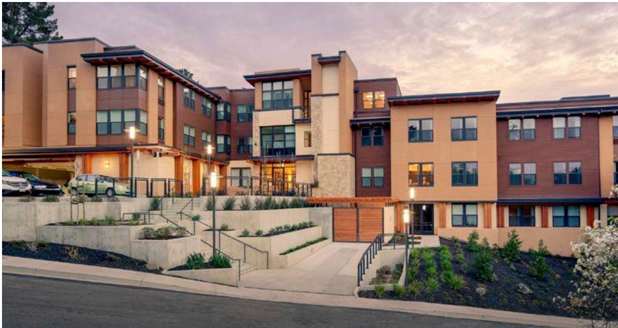
Eden Housing's Monteverde Senior Apartments | Orinda, CA | Designed by DAHLIN
