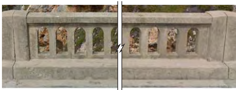
Original Barrier - Existing
