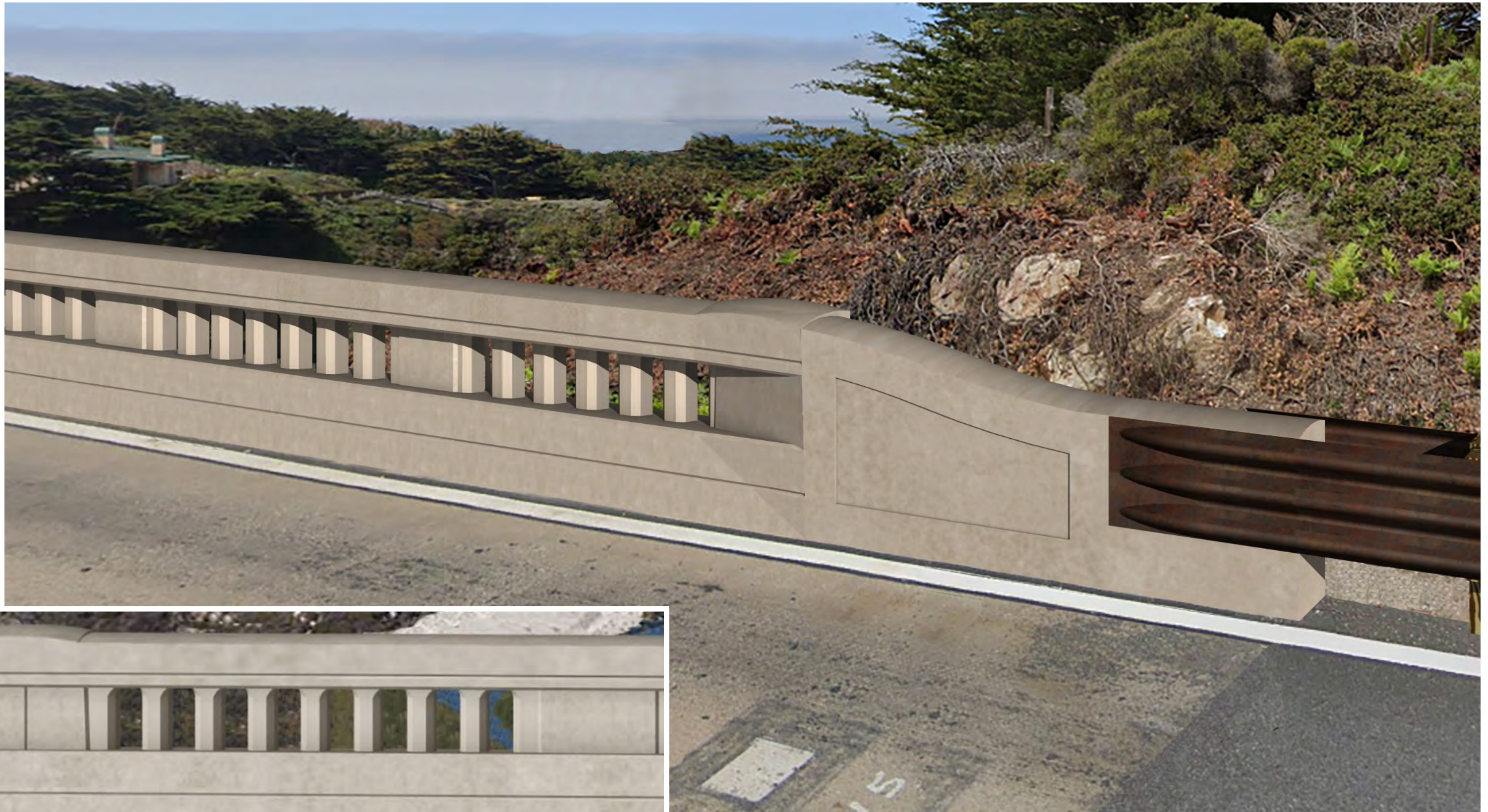
Barrier Alternative - 1 6" Clear Opening with Chamfered Balusters
