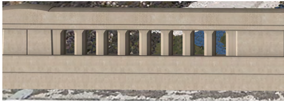
Barrier Alternative - 1 6" Clear Opening with Chamfered Balusters
