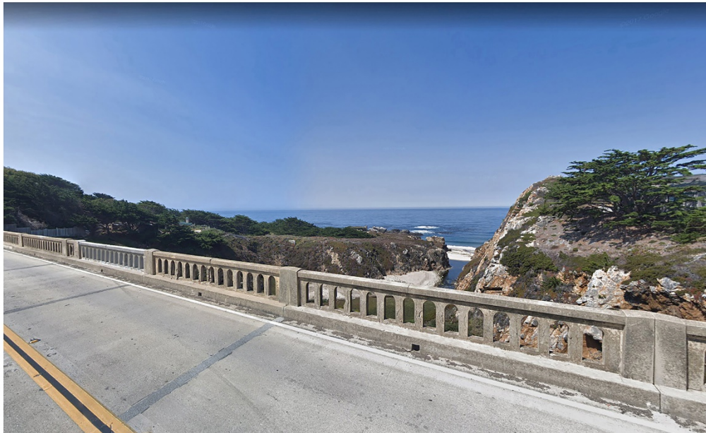
GARRAPATA BRIDGE EXISTING BARRIER
