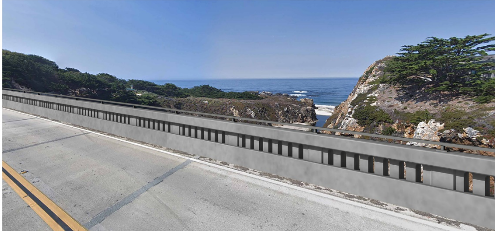
GARRAPATA BRIDGE BARRIER TYPE 86 PHOTO SIM.
