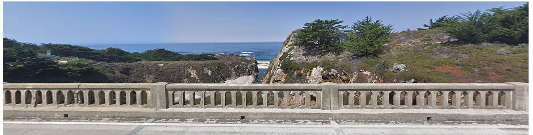
EXISTING ON DECK VIEW
