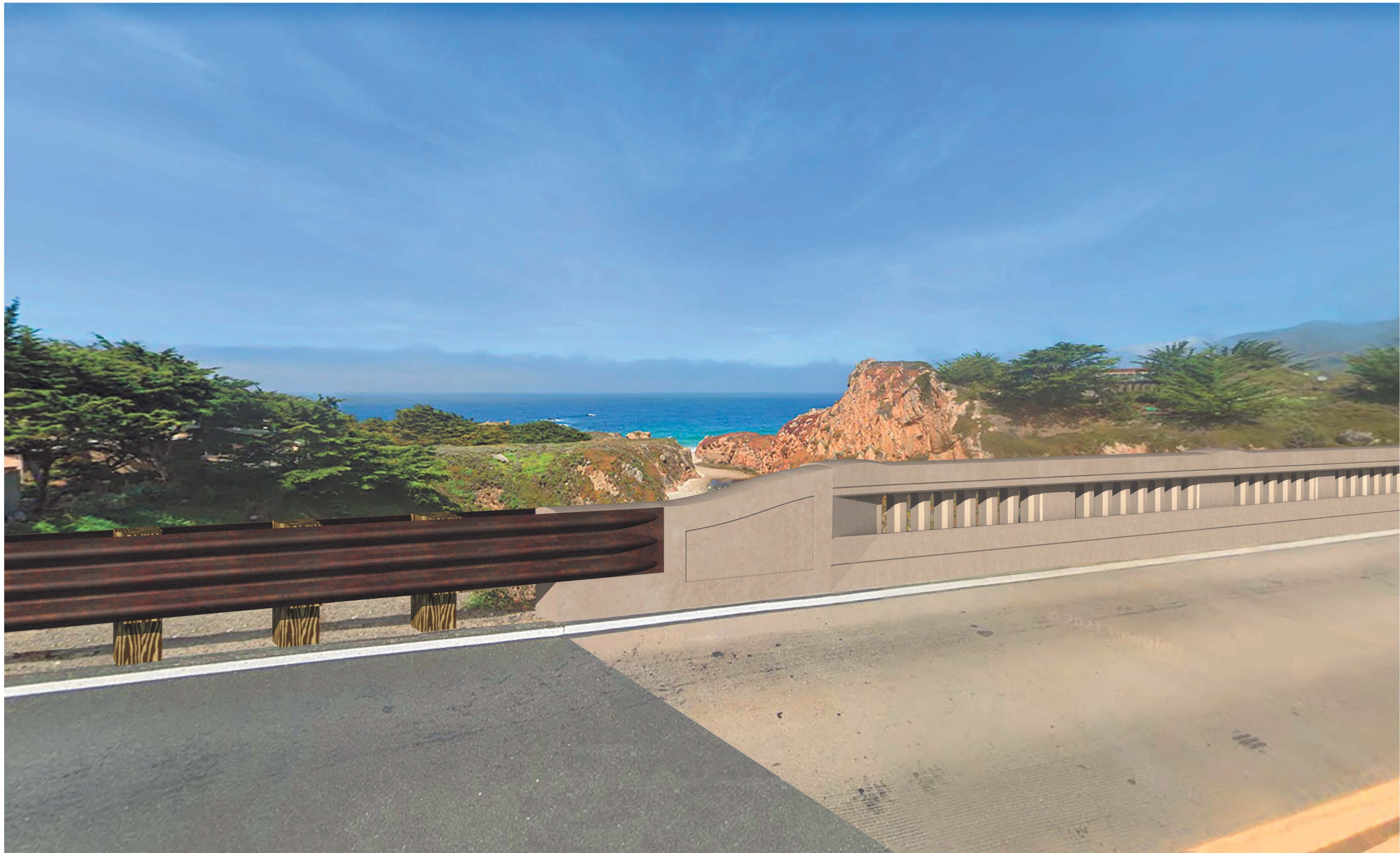
86H SOUTH END BLOCK PHOTO SIM.
