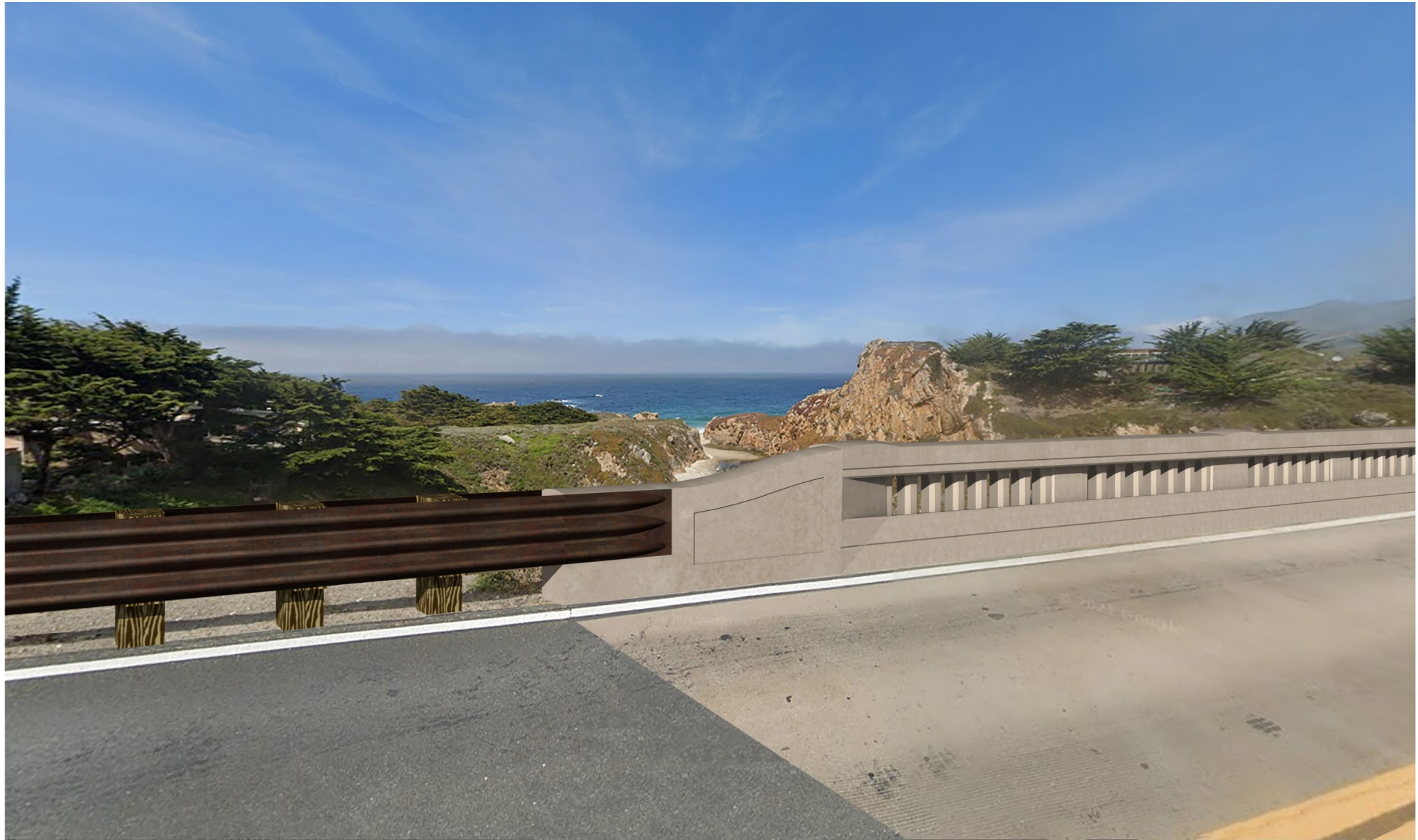
86H SOUTH END BLOCK PHOTO SIM.
