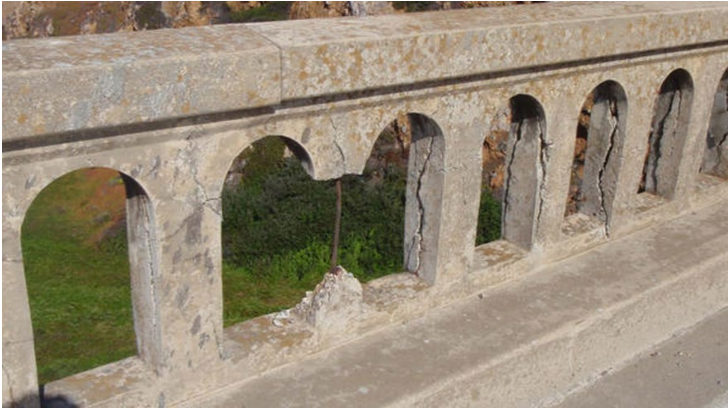
Existing photos of the Garrapata Creek Bridge
