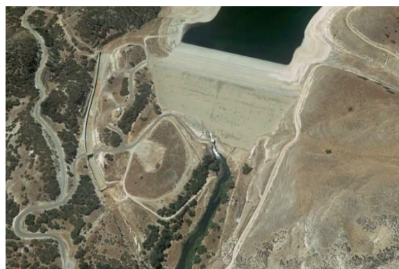
San Antonio Dam and Spillway
