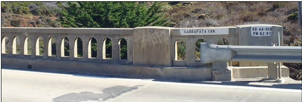
Garrapata Creek Bridge Rails, 2018
