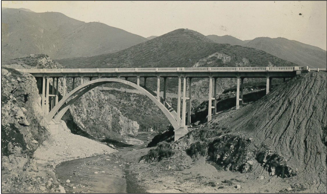
Garrapata Creek Bridge, February 1932
