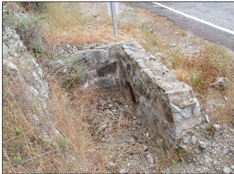
Contributing L-Shaped Masonry Culvert Headwall
