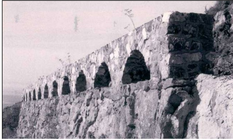
Arcade-style masonry parapet
