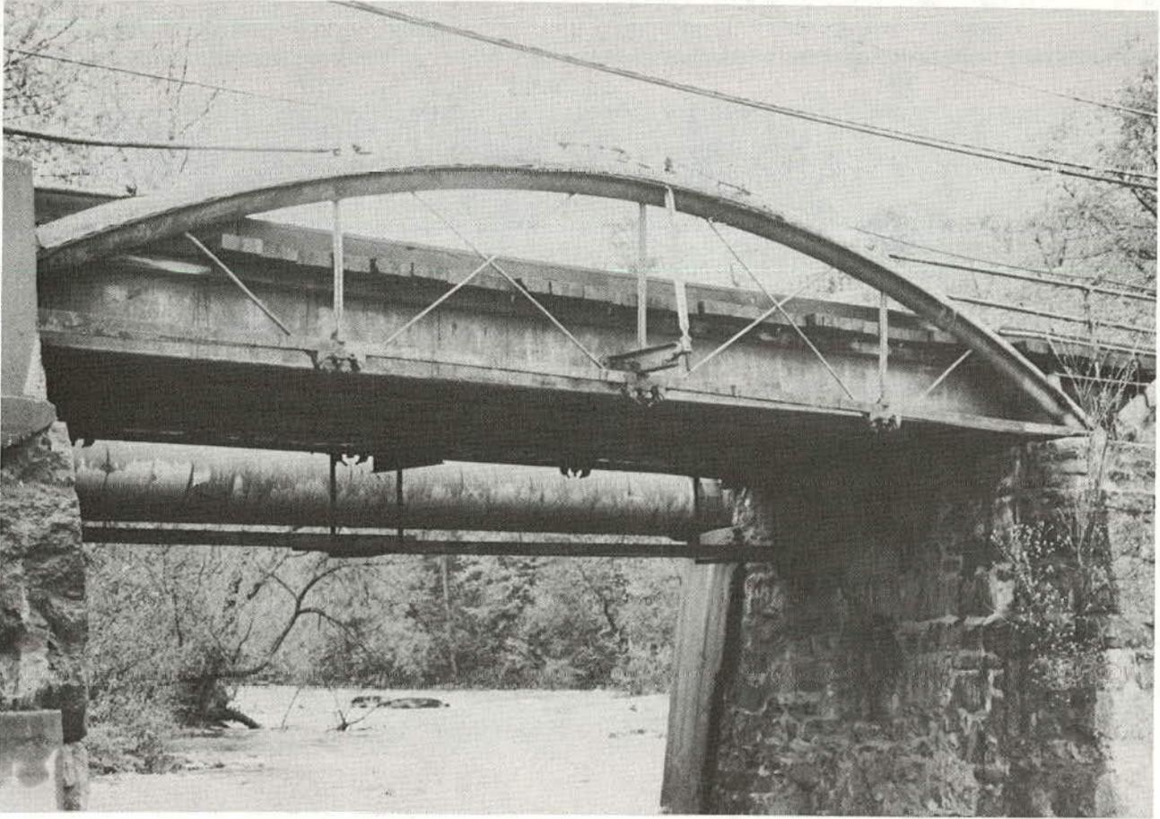
FIGURE 15 Trusses of the Tiaronda Bridge, Beacon, New York, built on the 1867 patent of Glass, Schneider, and Reznor, have been retained to delineate the replacement structure. (Photo by R. M. Vogel, Smithsonian Institution.)
