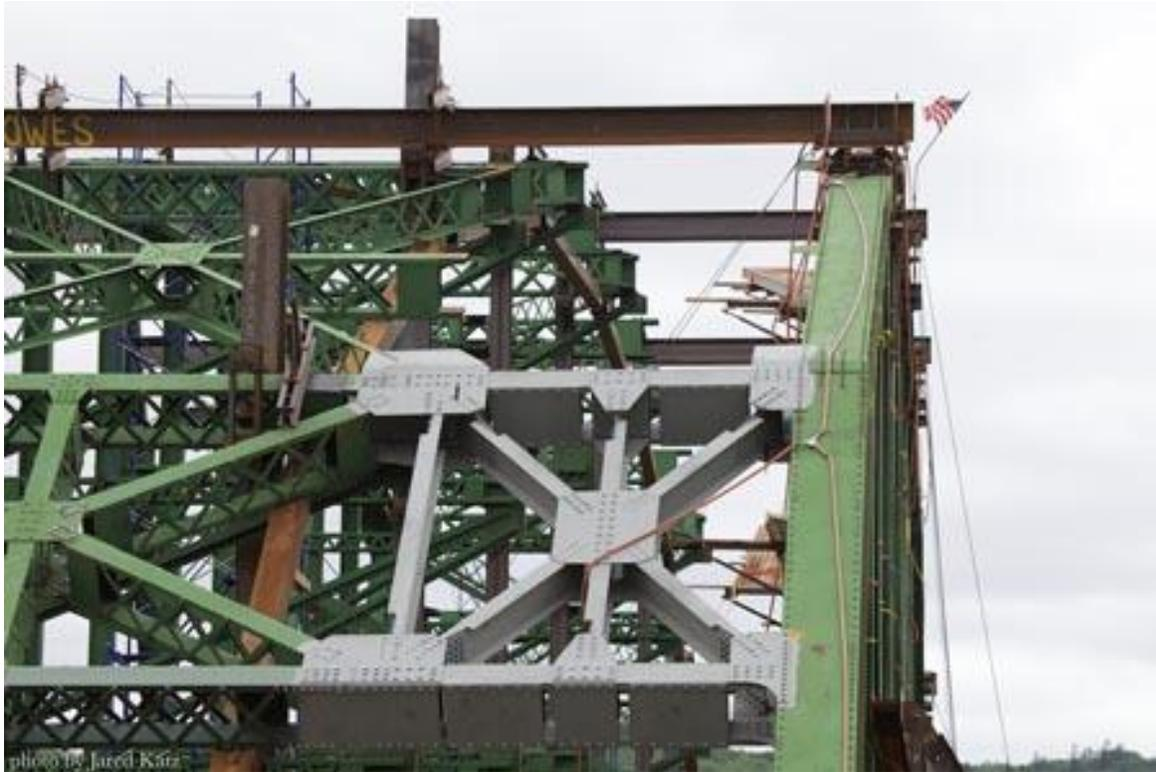
**Figure-11:** Checkered House Bridge with a new section of cross-bracing in place.
