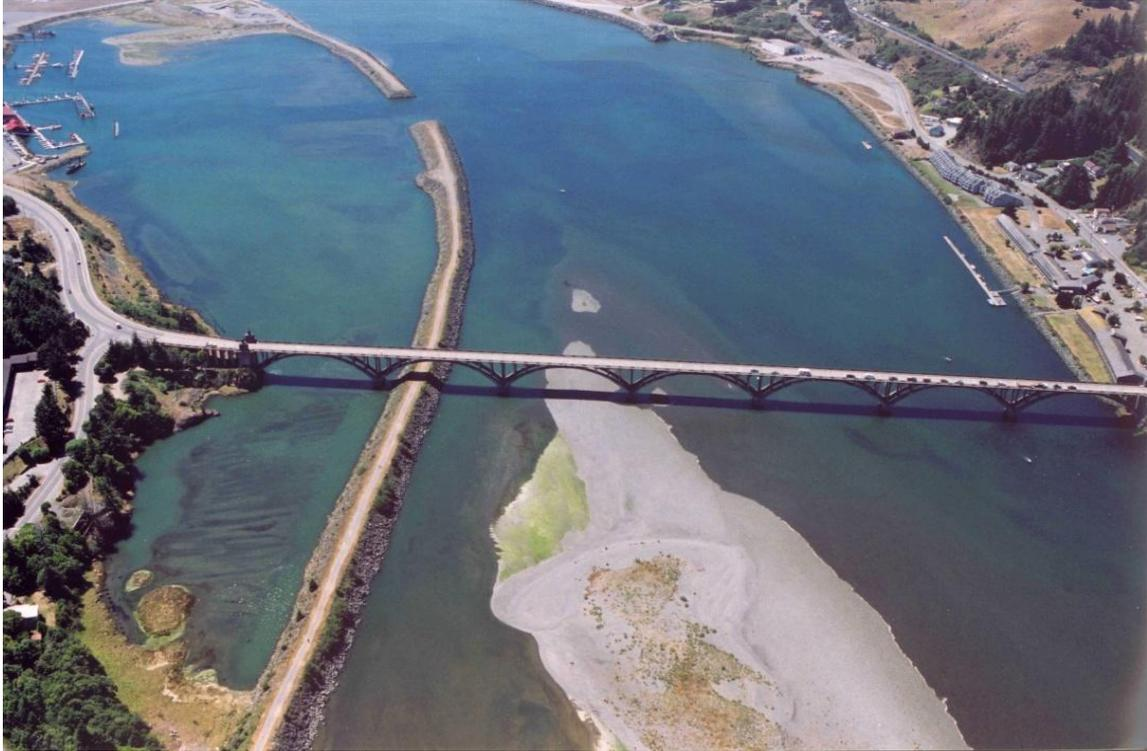
**Figure D-7:** The Rogue River Bridge (1931), Oregon, was rehabilitated with cathodic protection and a new deep foundation (Pier 1).
