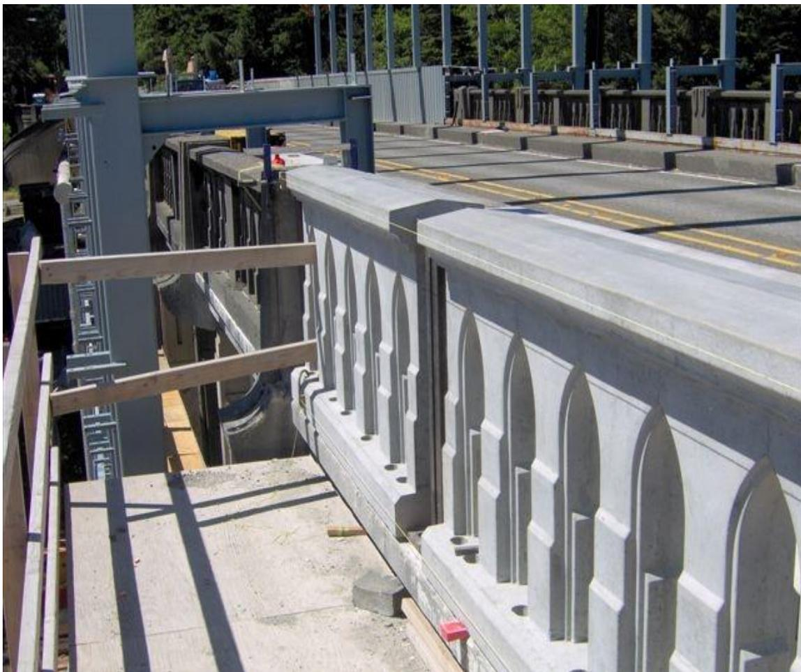
**Figure D-5:** A portion of the Coos Bay bridge rail (South Arched Section), in Oregon. The new stealth rail is in the foreground and the darker, original rail is shown in the background.
