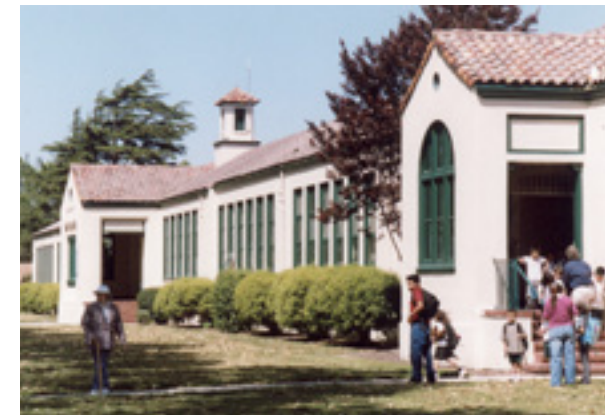
Even single-story buildings, when symmetrically arranged, can have a significant community presence.
