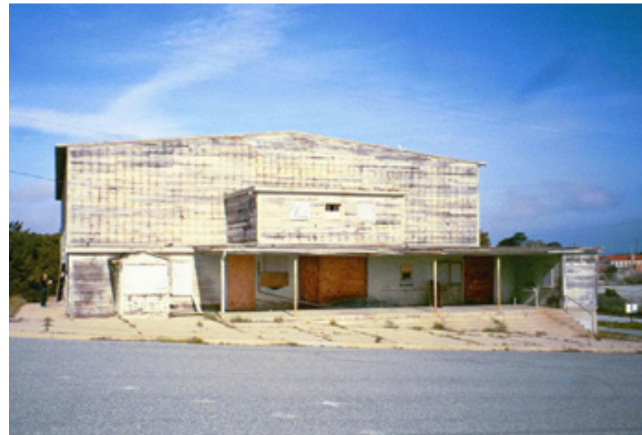
Theater elevation facing Sloat Street
