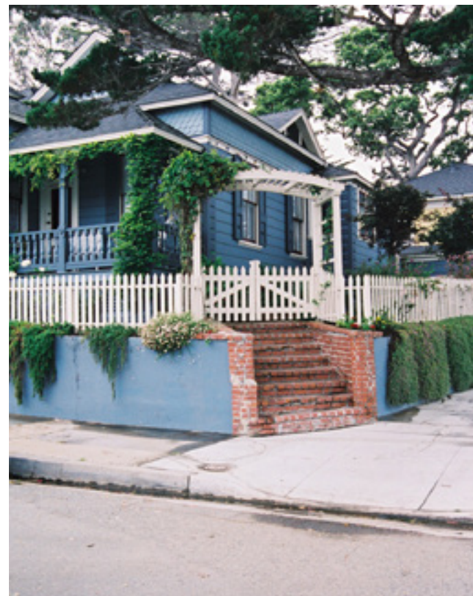
Stucco wall with fence
