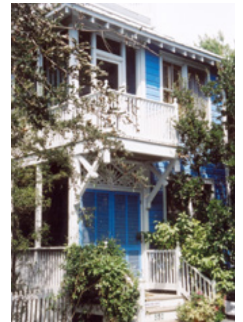
Craftsman porch details are structurally expressive.
