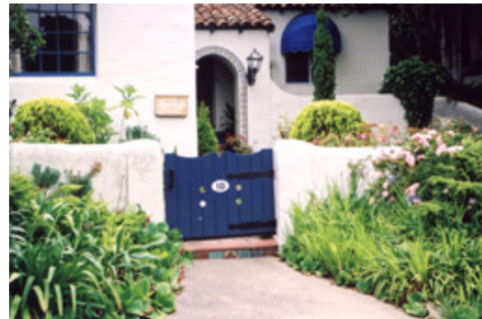
Stucco wall with gate
