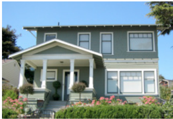
Asymmetrical window and door composition and a mix of siding materials are characteristic of the Garrison Craftsman style.
