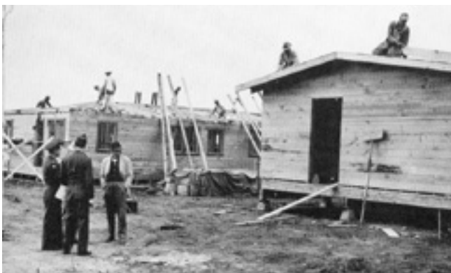
Figure 2.24 Construction at East Garrison circa 1940
