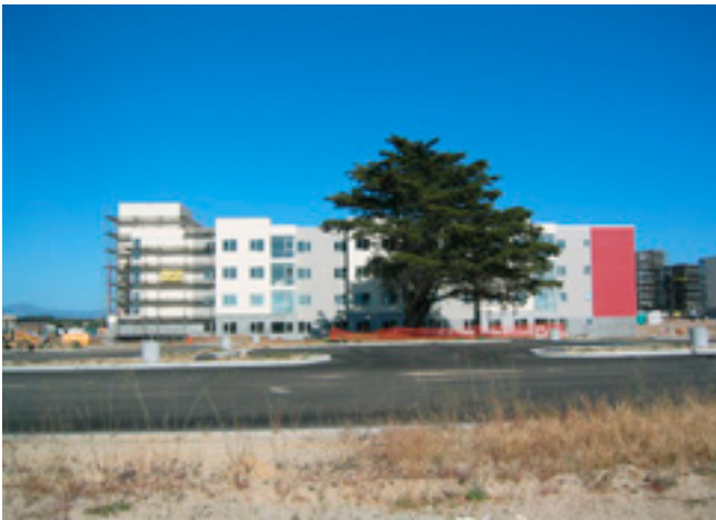
Figure 3.19 New construction at CSUMB
