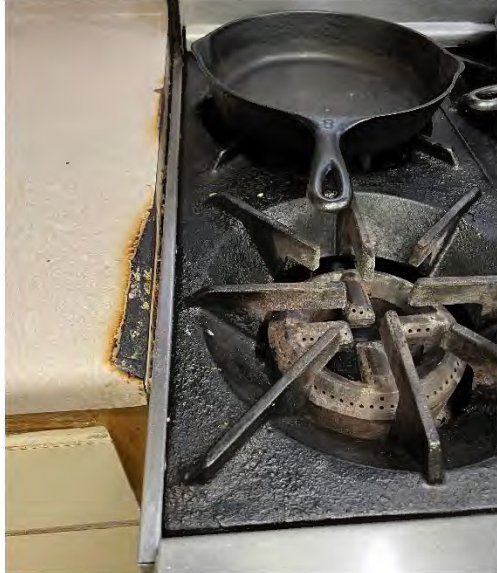
Old stove/counter top damage
