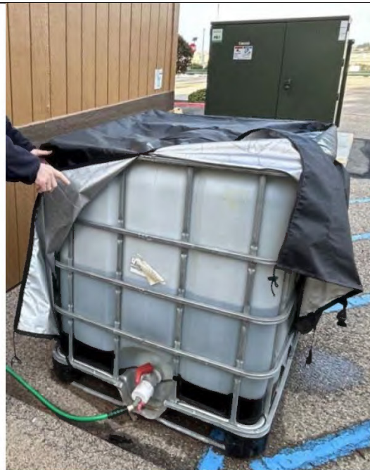
Non-potable water supply
