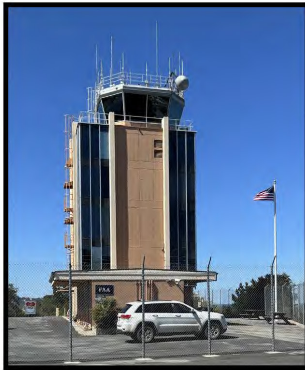
Monterey Regional Airport control tower. Photo taken by Civil Grand Juror.
