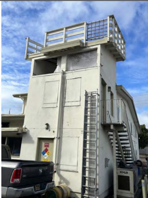
Abandoned training tower
