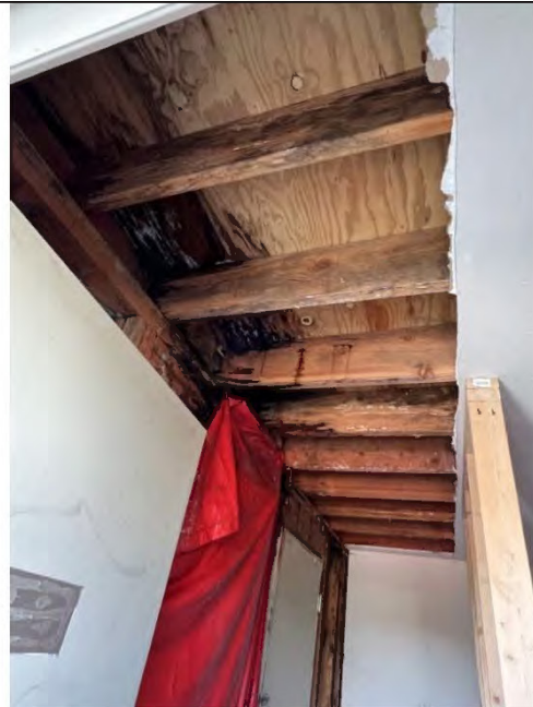
View inside abandoned training tower
