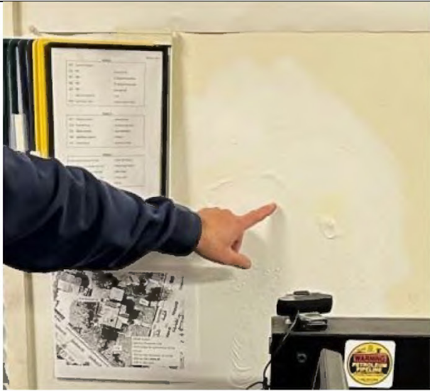
Bubbling paint after two weeks
