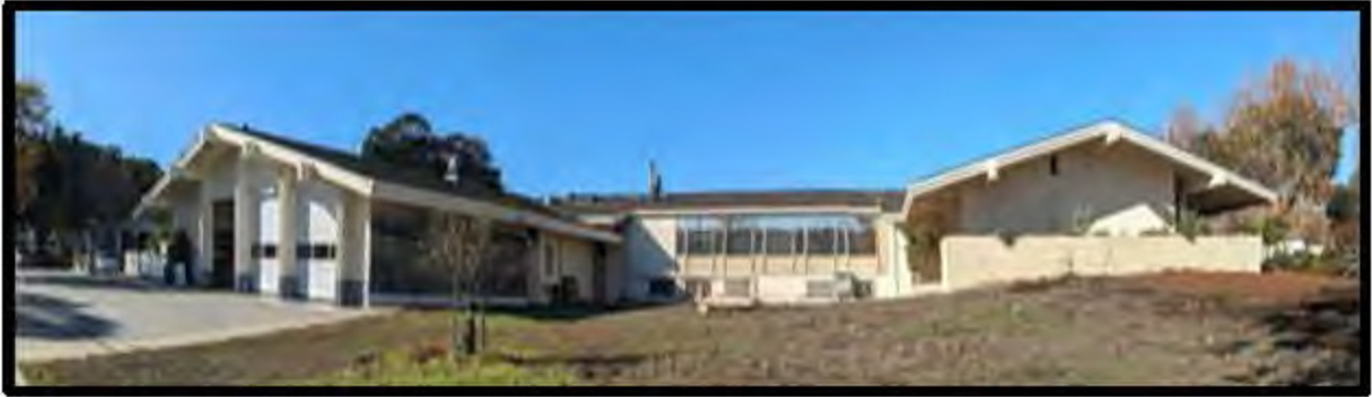
Downtown Monterey Fire Station 11 on Pacific Avenue Source: Photograph taken by Civil Grand Juror
