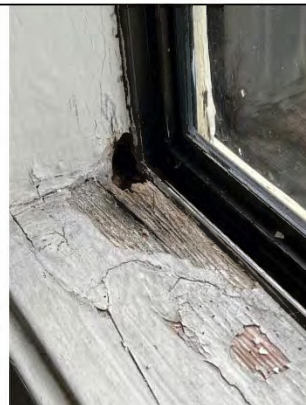
Kitchen area windowsill
