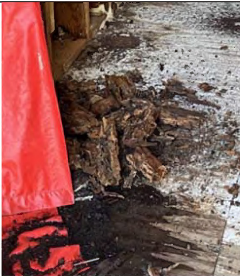
View inside abandoned training tower
