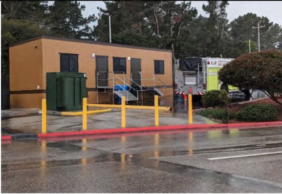
Modular trailer "fire station" at airport
