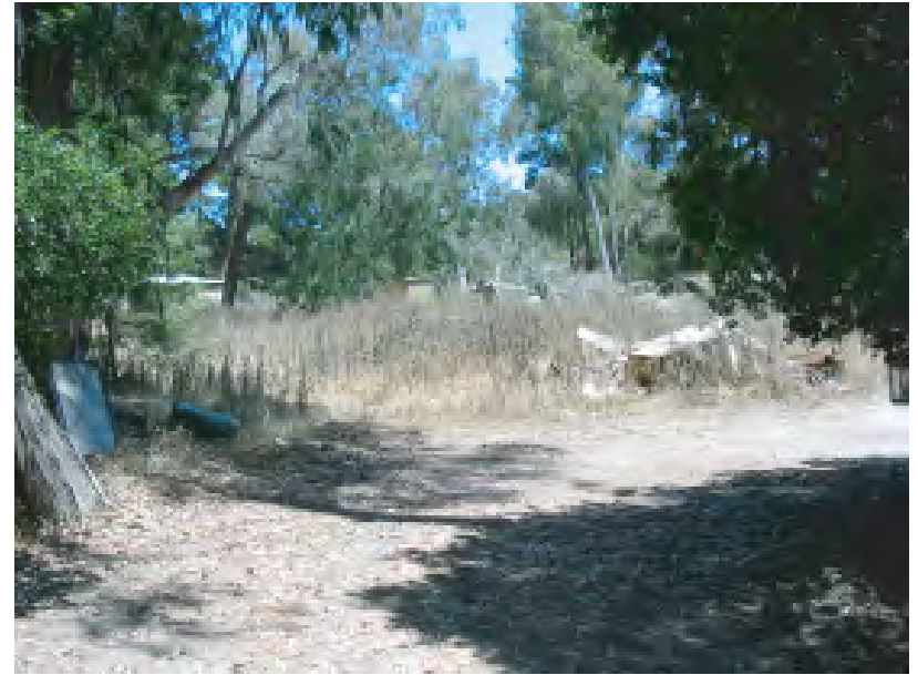
Photo 2. View of existing support structures and debris.
