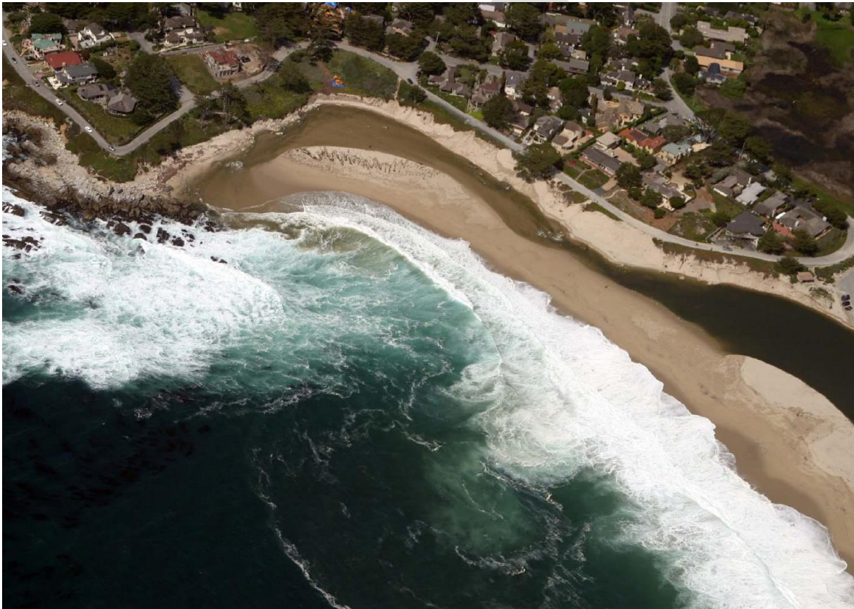
Figure 1-2 Example of lagoon migration north along the beach at the toe of the bluff carrying Scenic Road.
