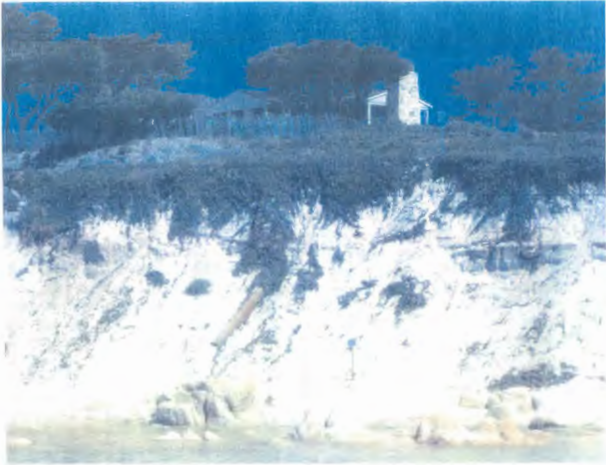
Figure 2: Scenic Road Coastal Bluff Showing Granite Bedrock at Base of Bluff 8/5/2005
