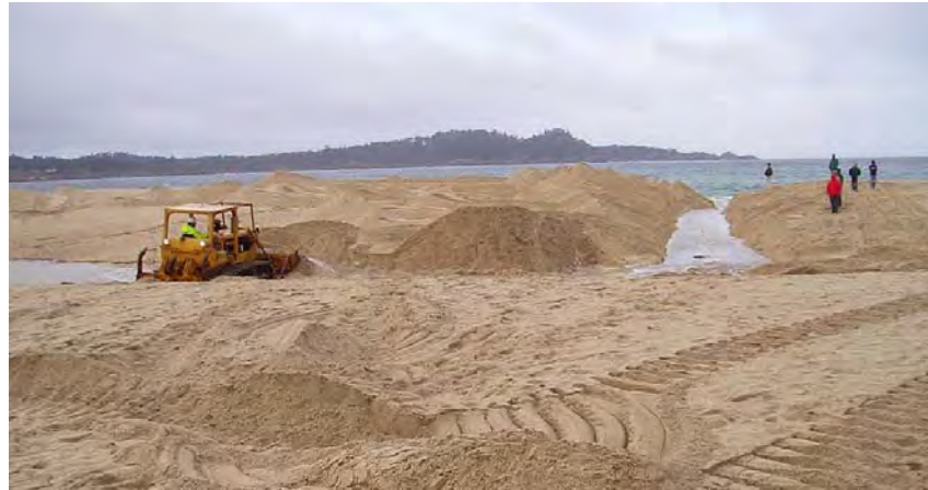
Cutting an outlet through the beach - December 2004
