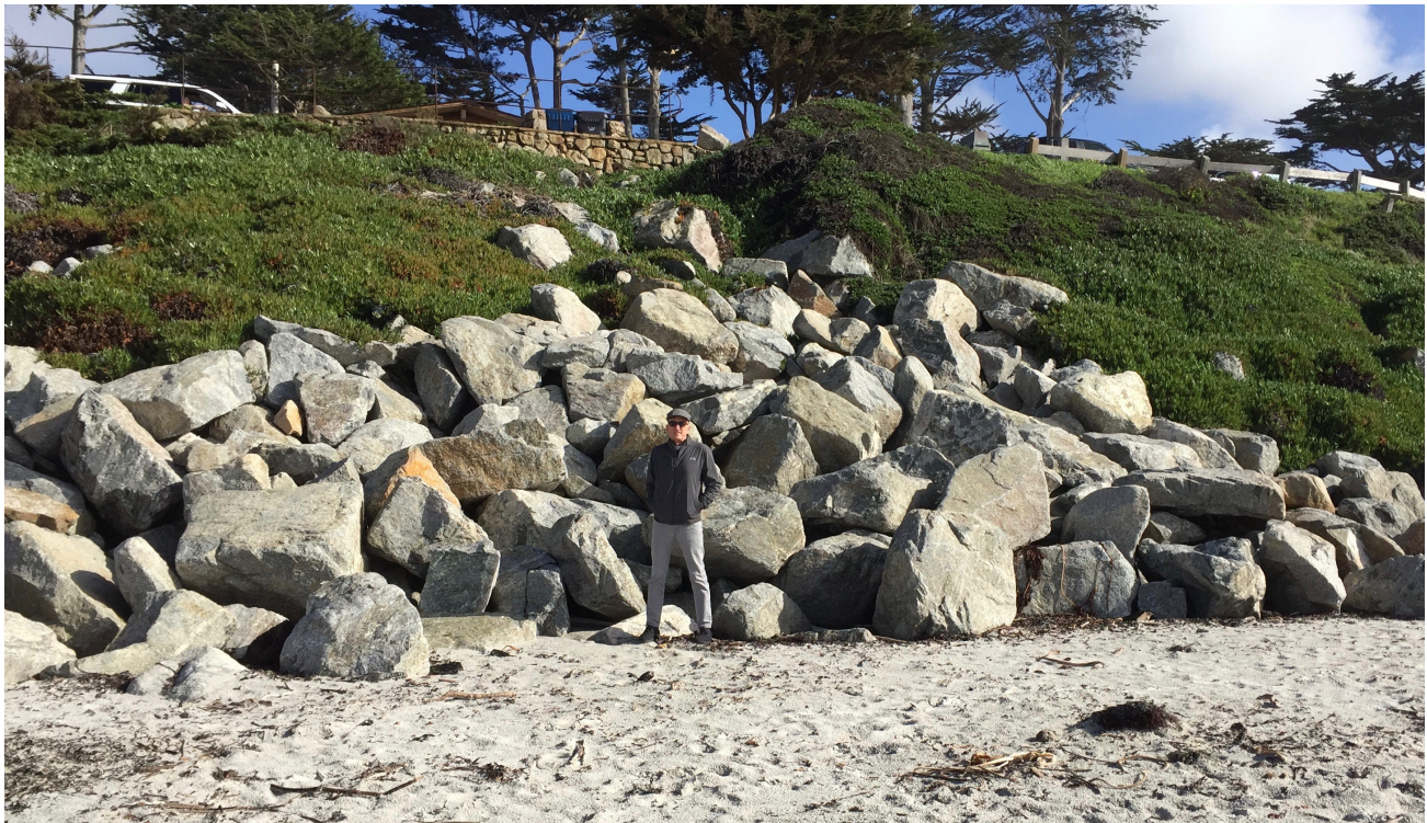
Rip-Rap at Carmel Beach - Is the material proposed for the SRPS?
