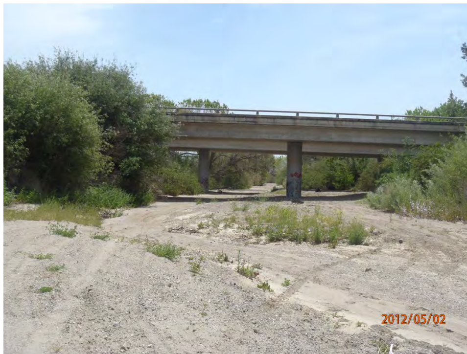
Photo 6. U.S. Highway 101 Overpass within San Lorenzo Creek
