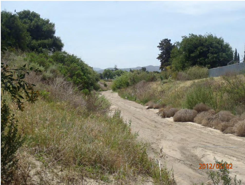
Photo 5. Looking Upstream into San Lorenzo Creek from the Confluence with the Salinas River
