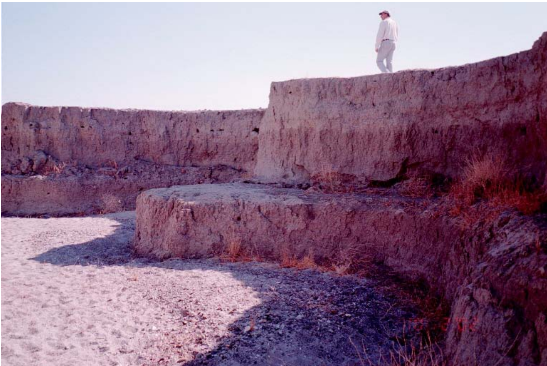
Photo 4.3 Cholame Creek bank erosion. This creek is one of the sources of sediment in the Salinas River.
