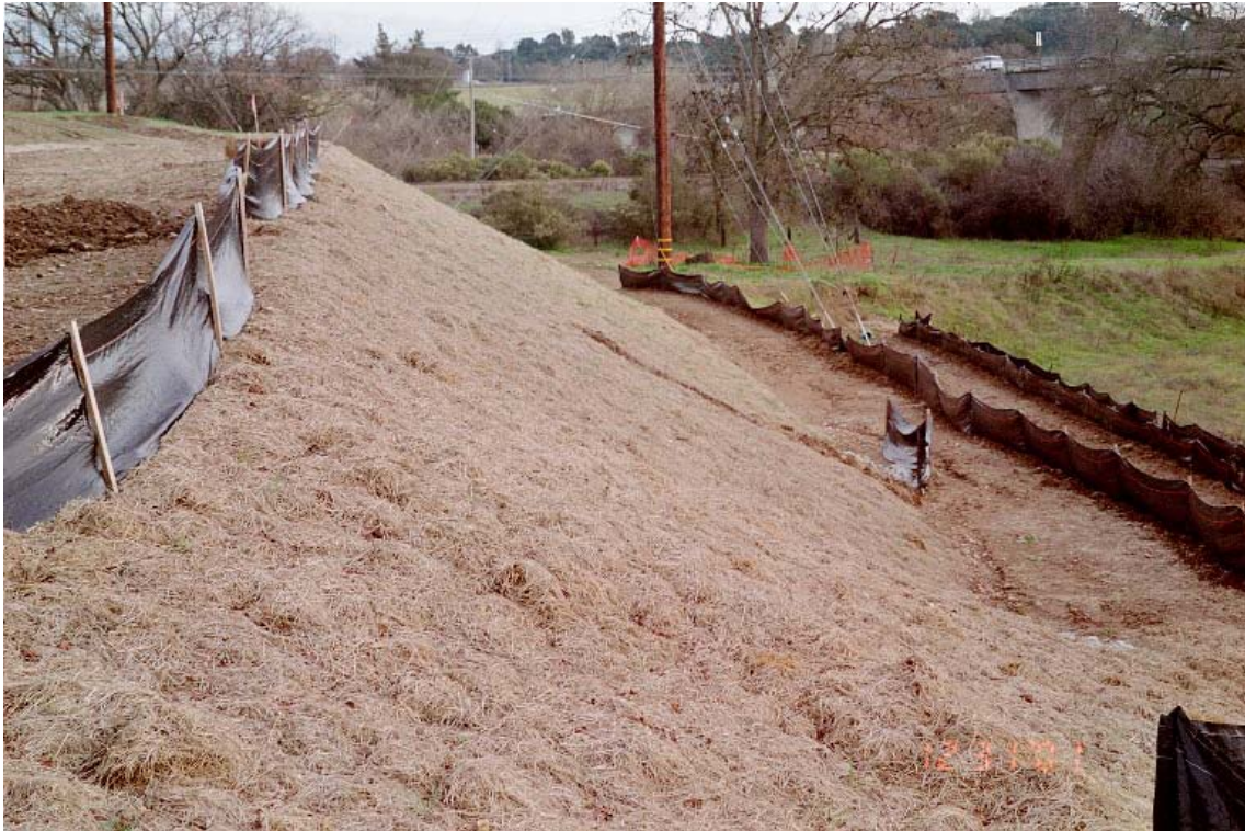
Photo 7.9 Example of good erosion control implementation measures.
