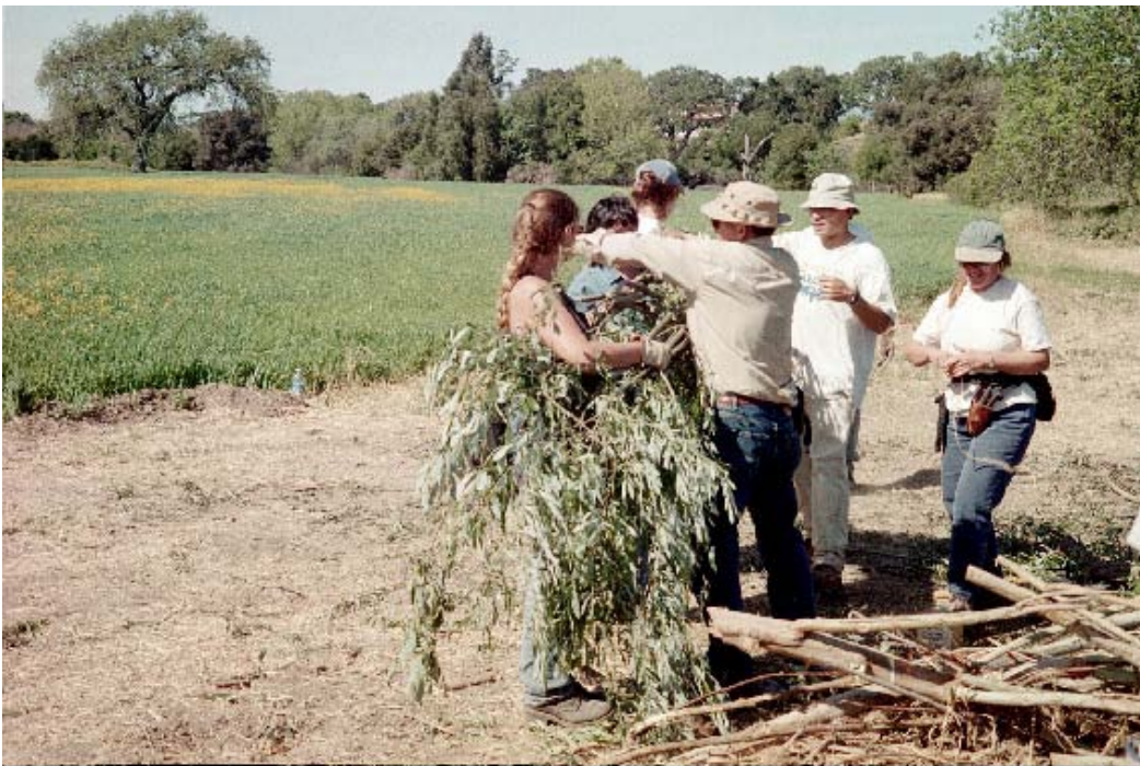
Photo 7.7 NRCS instructs US-LT RCD and others in the construction of willow wattles and other bioengineering techniques of stream channel restoration
