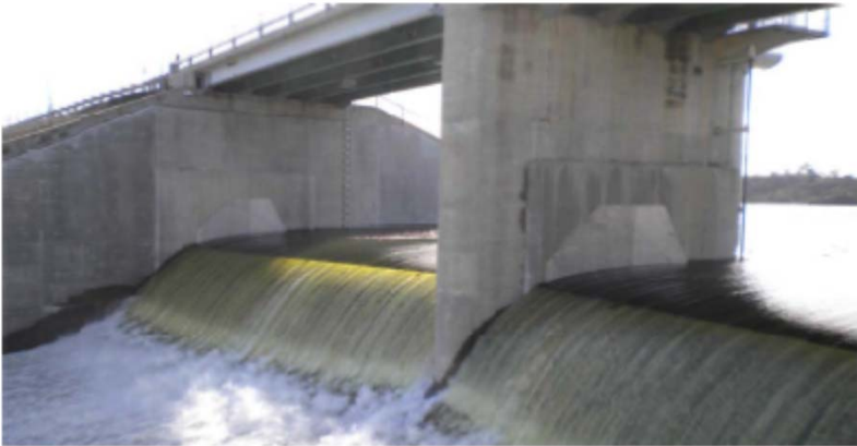
Figure 6: Spillway Modification to Nacimiento Dam
