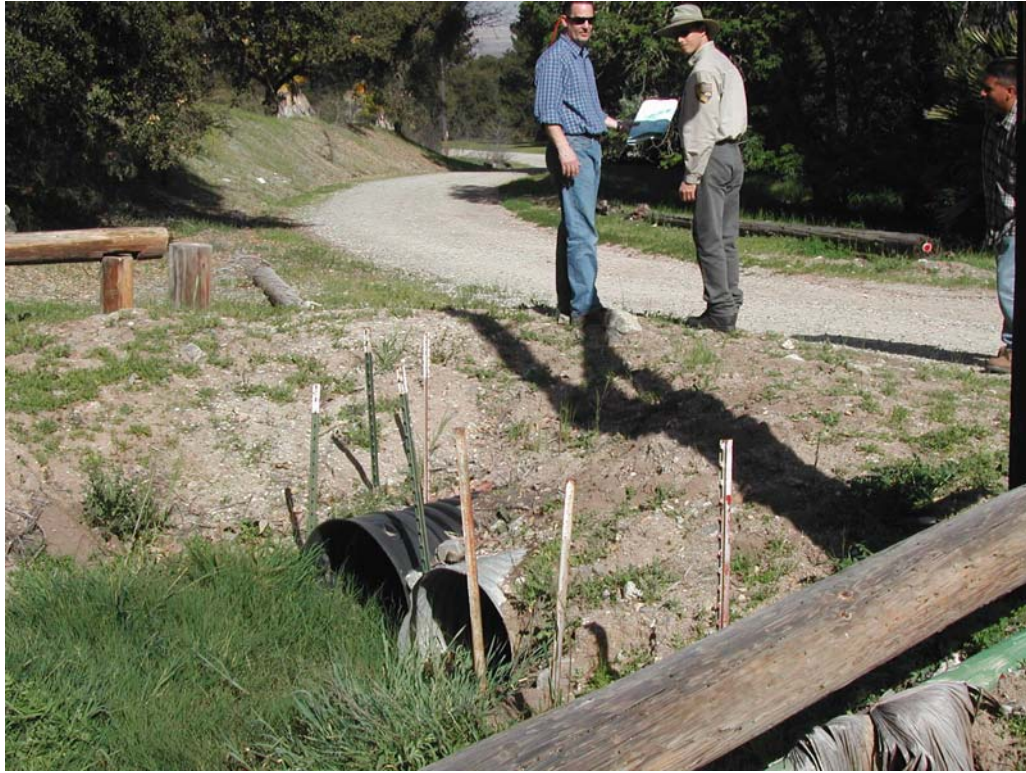
Photo 1: Existing culverts on the Project Site above the eastern property line
