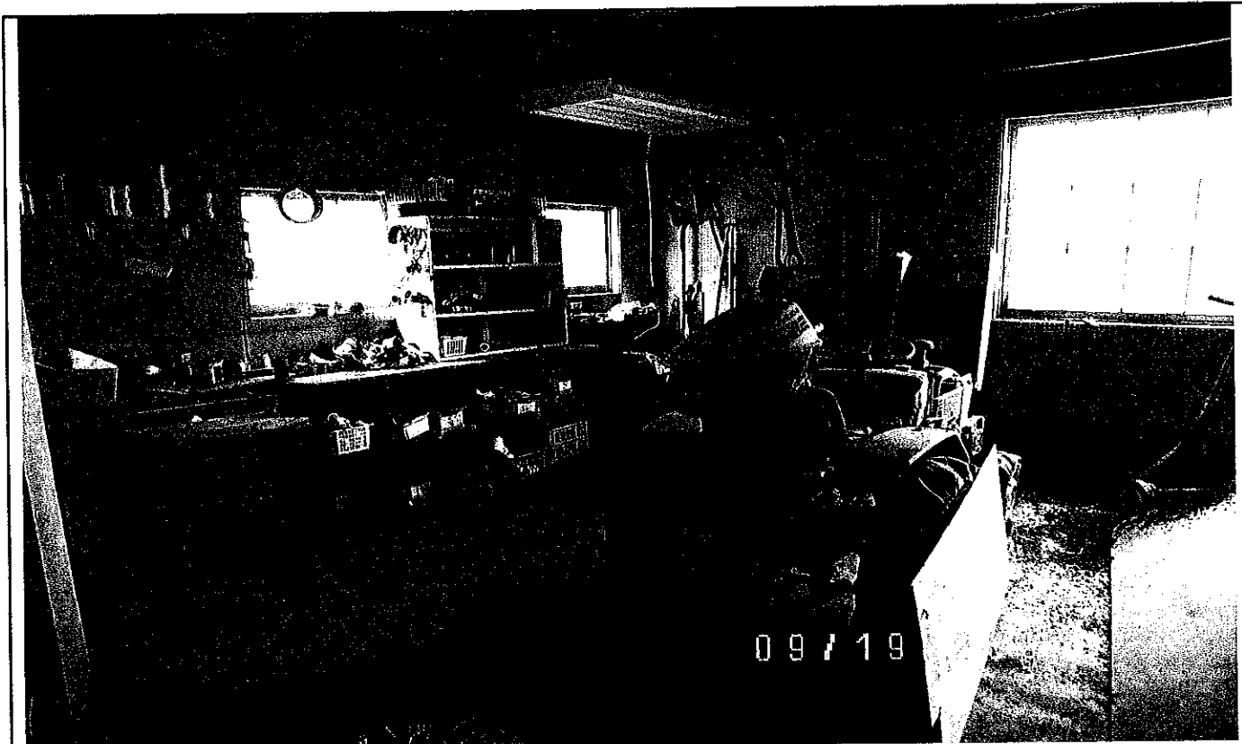
19. INTERIOR VIEW OF SHOP. NOTE HANGING FLOURESCENT FIXTURE.
