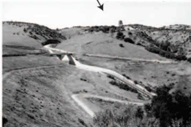
Spillway chute (looking north)
