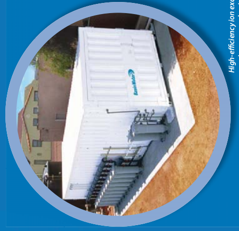
High-efficiency ion exchange nitrate removal unit
