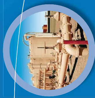
High-efficiency ion exchange nitrate removal unit
