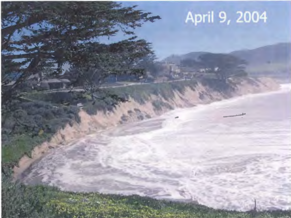
Figure 1: April 9, 2004 Photograph showing Scenic Road, the Eroding Coastal Bluffs Below, and Beach Inundation from the Pacific Ocean (Thornton, 2005)
