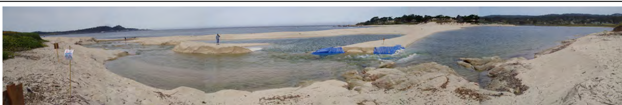
Temporary sandbags and tarps were used to raise the lagoon water level in Summer 2006
