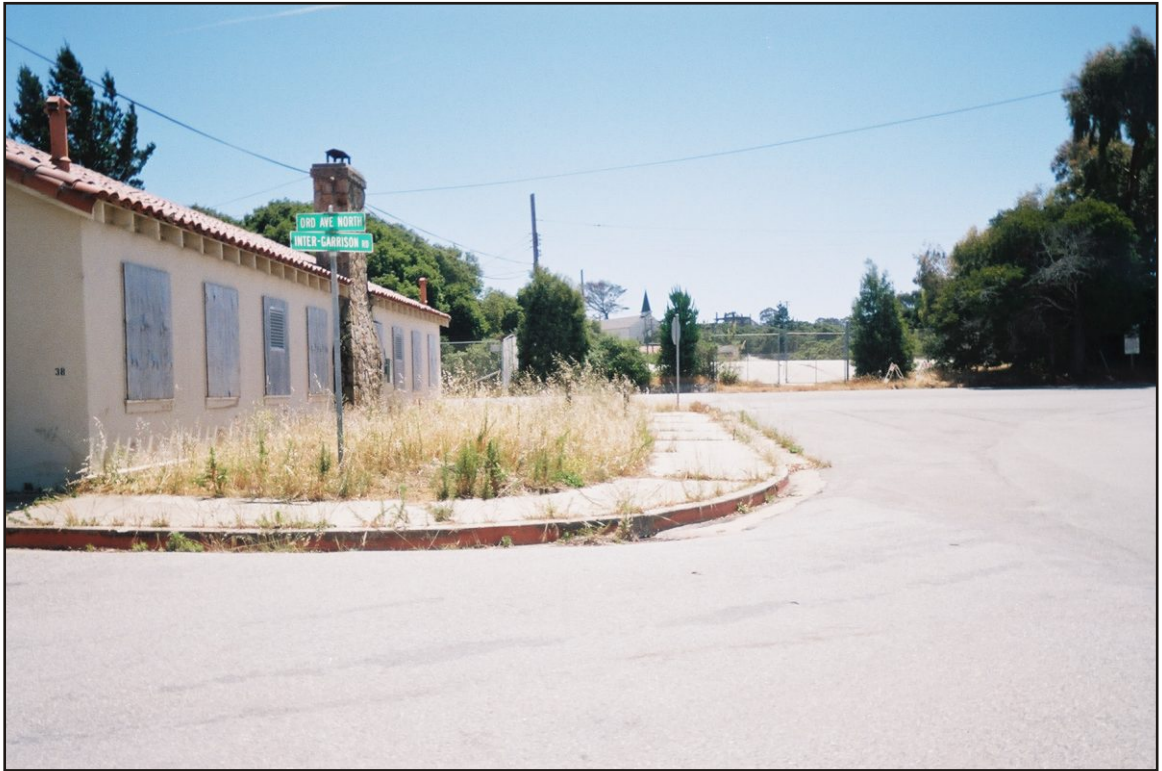
Photograph 1: View from Ord Avenue and Inter-Garrison Road looking south.
