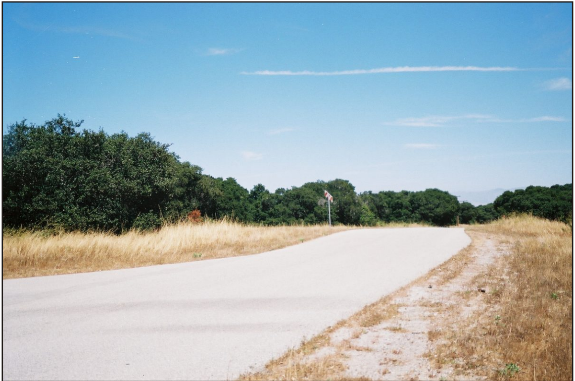
Photograph 6: View from Watkins Gate and West Camp Road looking east.
