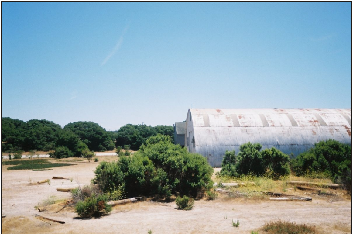
Photograph 8: View from center of project site looking southeast.
