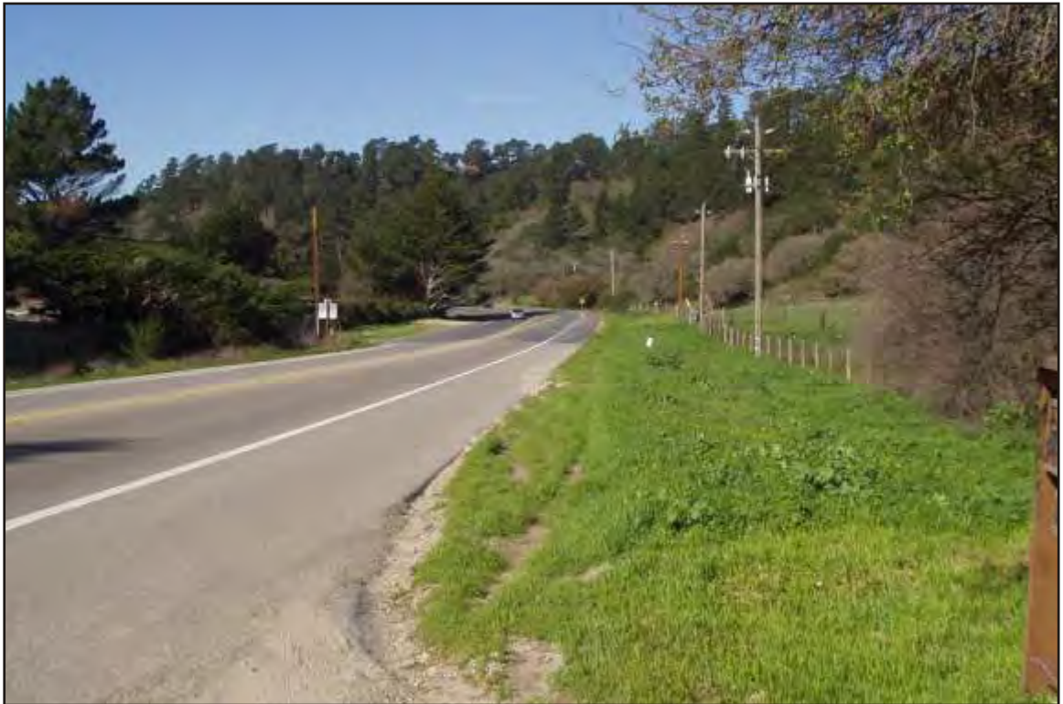
Photograph 8: Looking west down Carmel Valley Road from existing access drive.
