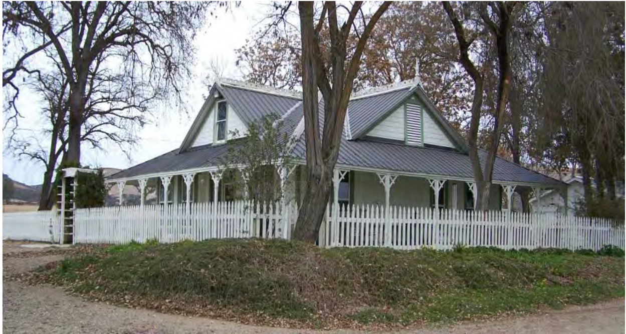
Figure 34. Current view of the Patterson Adobe. (Photo taken by Galvin Preservation Associates Inc.)
