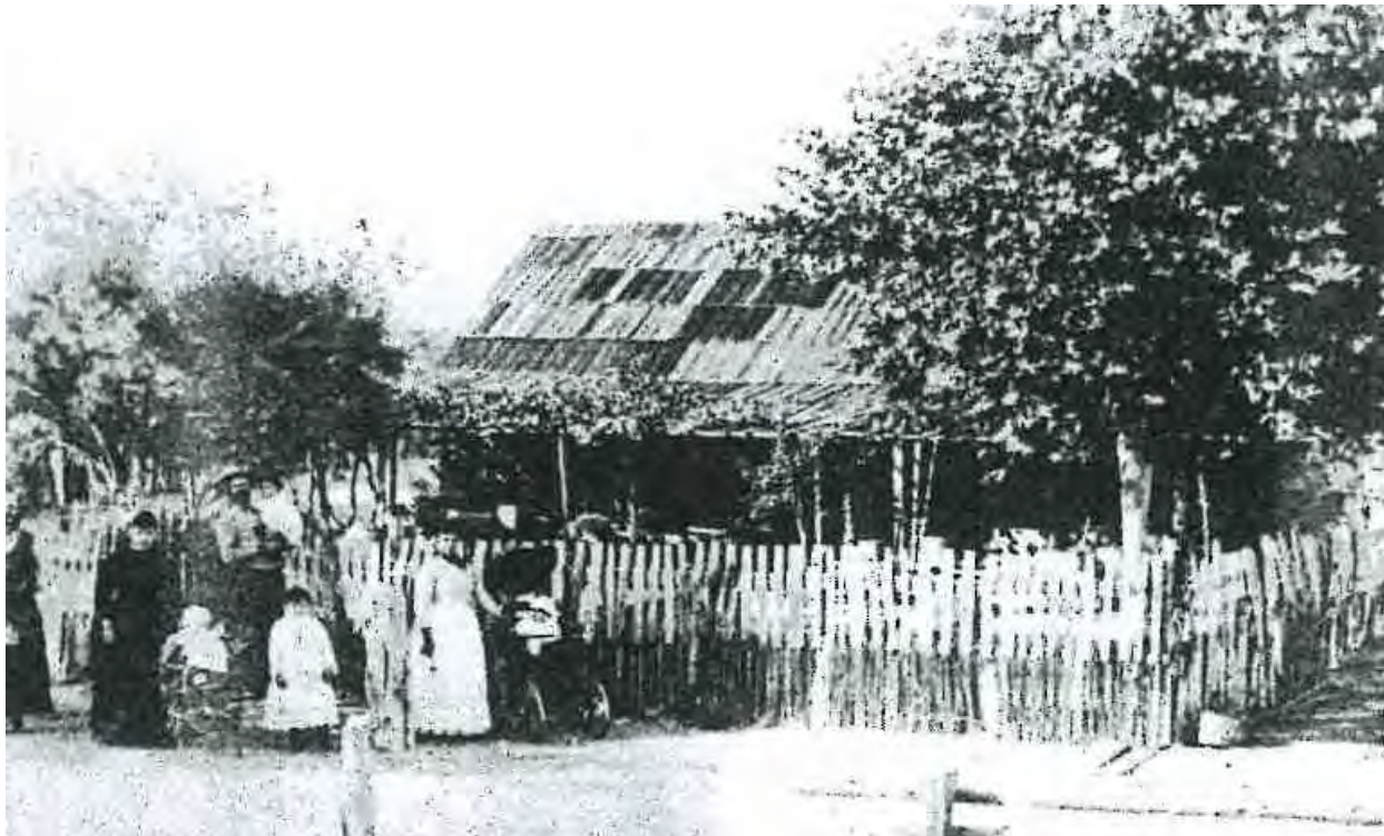
Figure 29. Photo of Cruz Diaz Adobe. It is constructed in the typical Spanish adobe style with a side gabled roof and a porch under a shed roof. (From Lost Adobes of Monterey County by Don Howard, p. 42)
