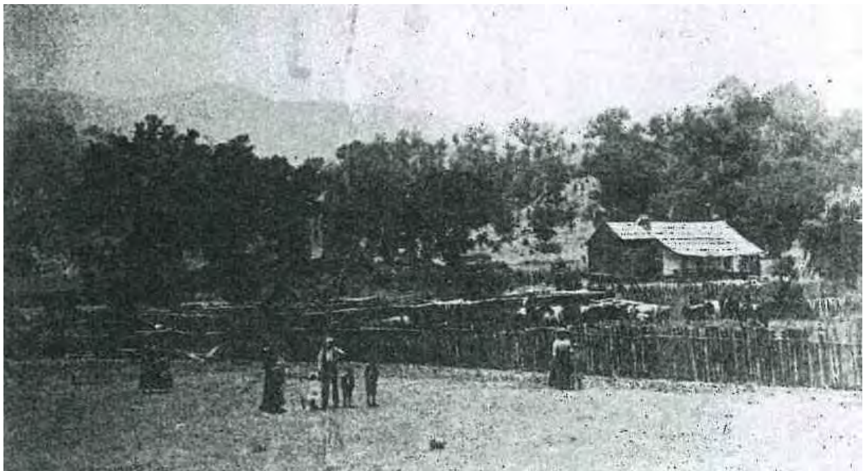
Figure 30. View of the Job Wood Adobe with its associated picket corrals. This is a typical scene of an early homestead from the 1860s and 1870s. (From "Lost Adobes of Monterey County" by Don Howard, p.99).
