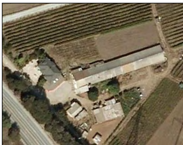
The Snyder Ranch at 1875 San Juan Road retains a packing shed behind the house, as well as other outbuildings. (Courtesy of Google Earth, 2007.)
