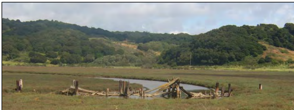
Remnants of timber pile foundations from Hudson's Landing. (PAST photograph, 2010.)
