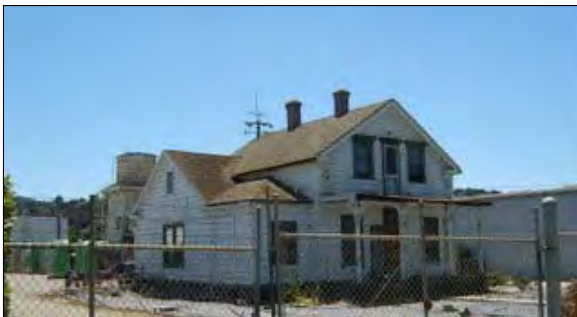
At 1372 San Juan Road, the Greek Revival house and tank house are the only historic buildings on the property. (PAST photographs, 2010.)
