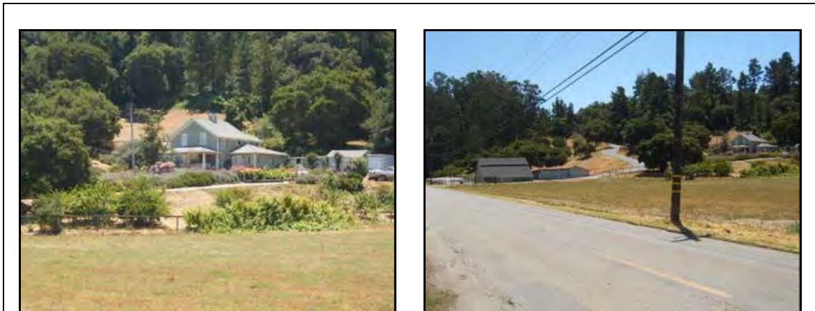
Views of Hutchings Ranch, 350 San Miguel Canyon Road. (PAST photographs, 2010.)
