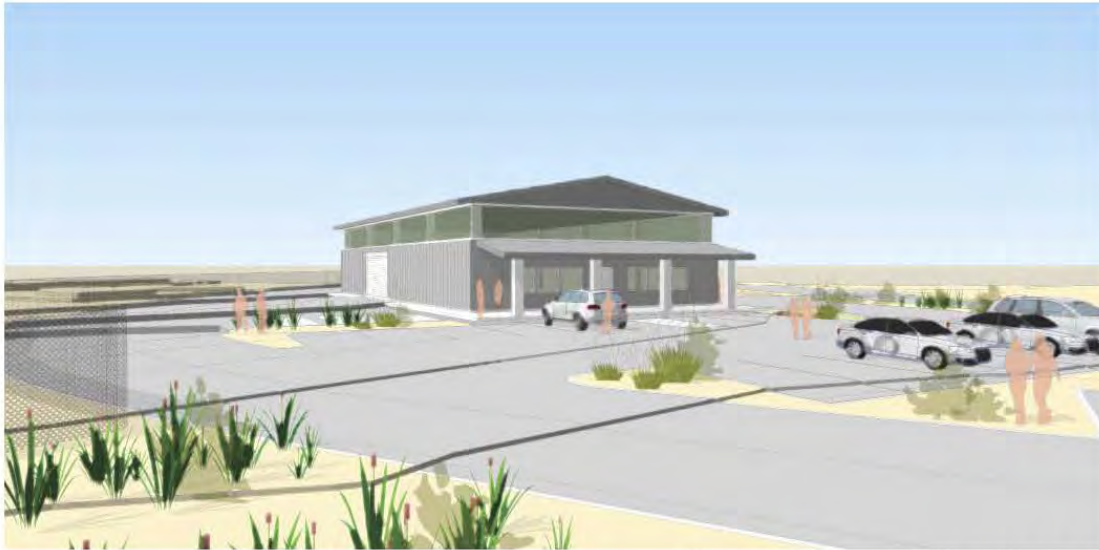
view 1 from sandholdt road
