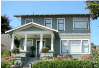
Asymmetrical window and door composition and a mix of siding materials are characteristic of the Garrison Craftsman style.
