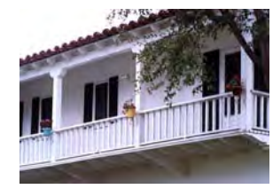
Exposed rafter tails add character to Mediterranean Revival eaves.
