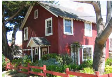
Simple forms with exposed structural members and deep overhangs are typical.
