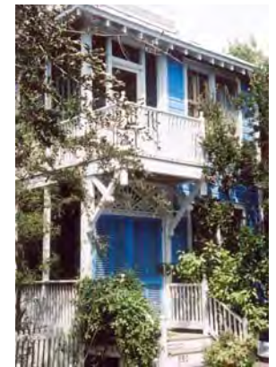
Craftsman porch details are structurally expressive.
