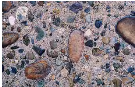
Exposed aggregate concrete paving
