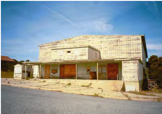
The simplicity of porches at the East Garrison is reflective of the utilitarian nature of the East Garrison buildings and should be maintained.
