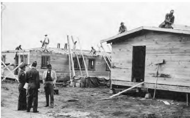
FIGURE 2.9 Construction at East Garrison circa 1940
