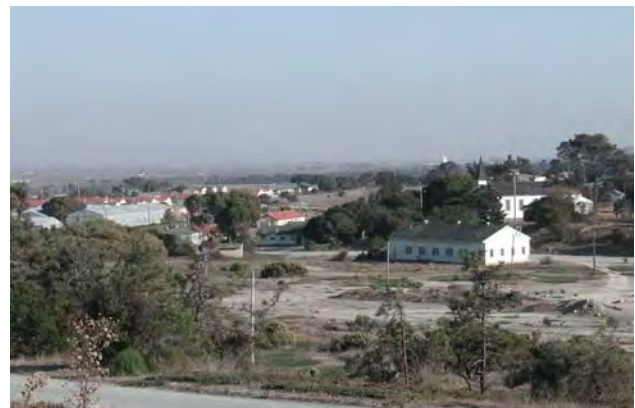
FIGURE 1.4 Abandoned buildings at East Garrison
