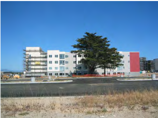
FIGURE 3.19 New construction at CSUMB
