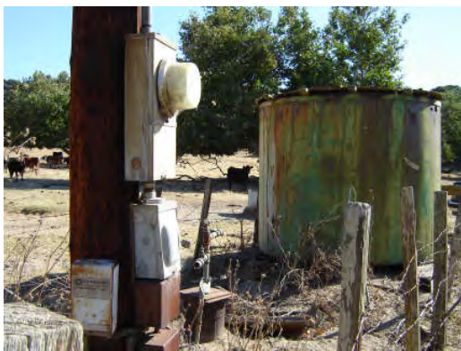
Apparently abandoned groundwater well on grazing part of southern portion of site
