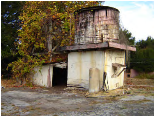
Old water tower and associated structure
